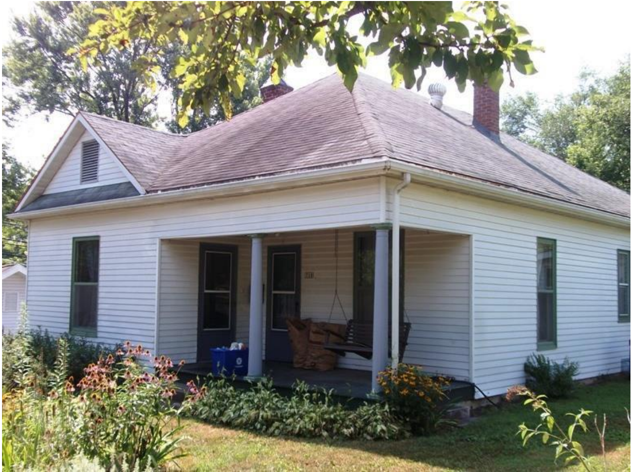
Figure 10. Blair family house constructed by James N. Blair – 715 W. 13 th Street – Contributing Architectural Style: Pyramid Roof Cottage (c. 1900)
