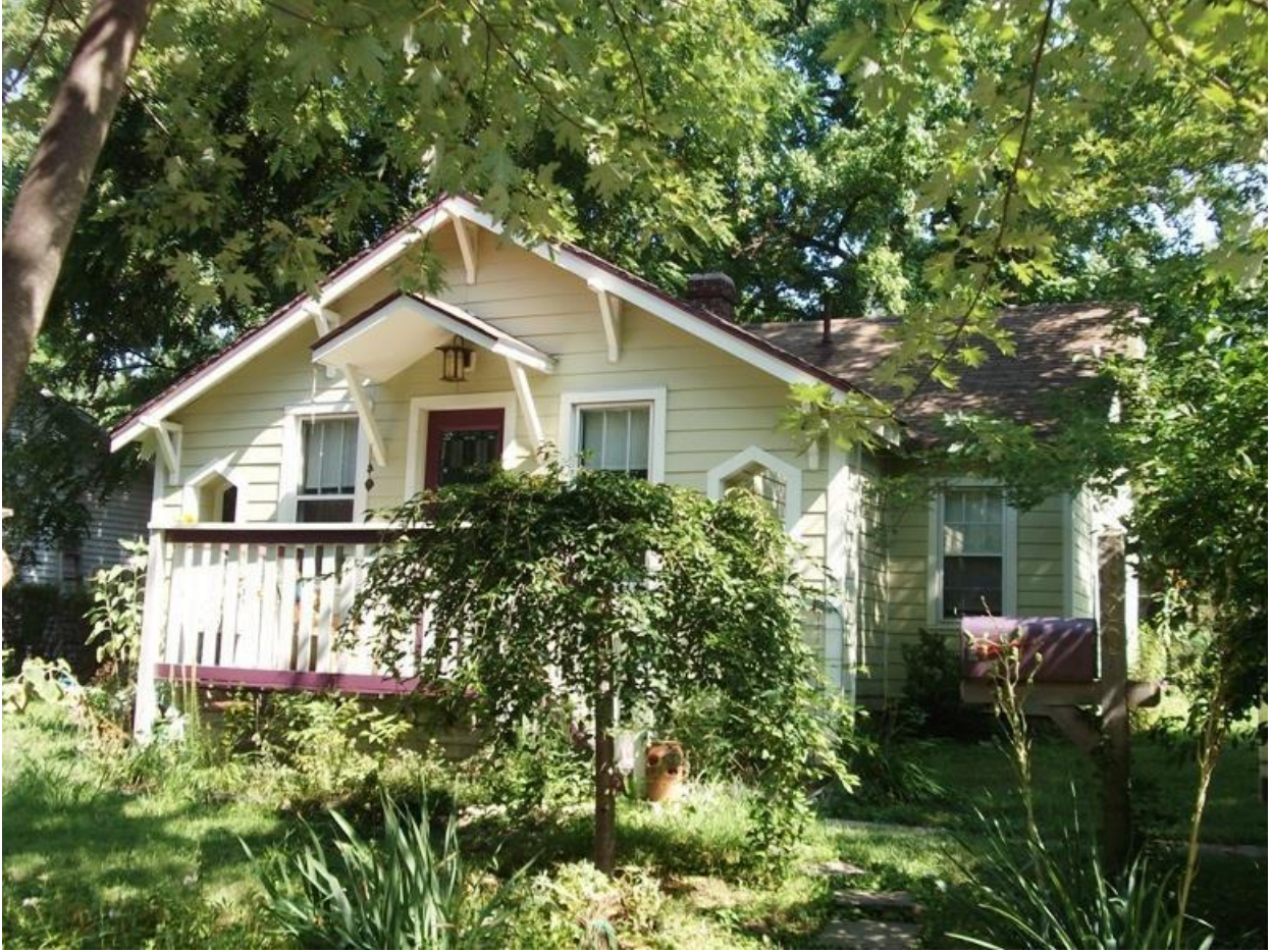
Figure 19. 600 W. 12 th Street – Contributing Architectural Style: Gable Ell (c. 1930)
