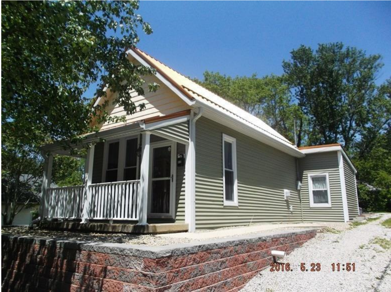
Figure 14. 612 W. 12 th Street – Contributing Architectural Style: Shotgun
