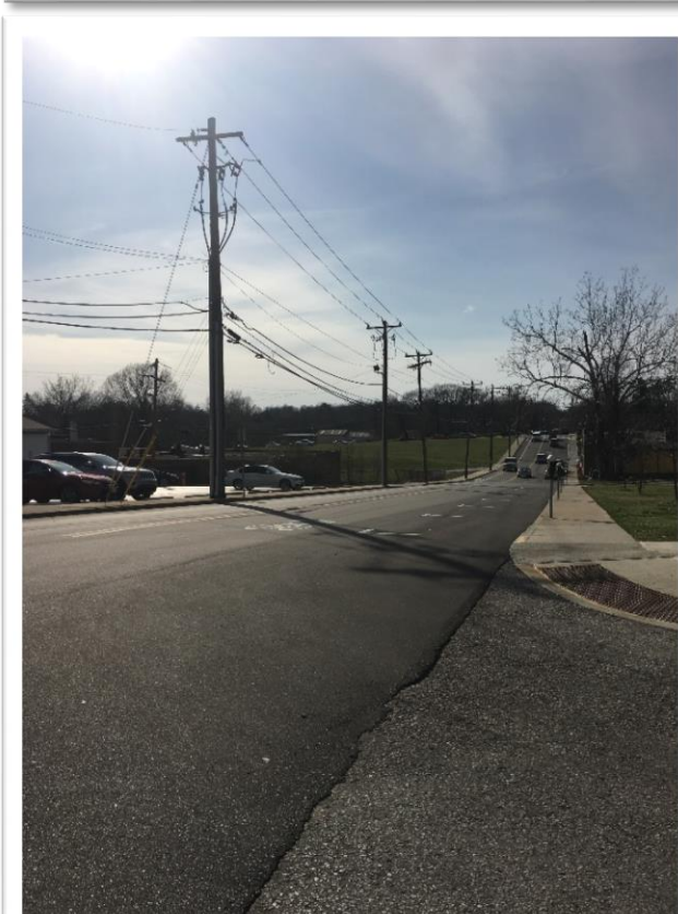
Current drivers' line of sight looking west at 11th St traveling south on Morton St
