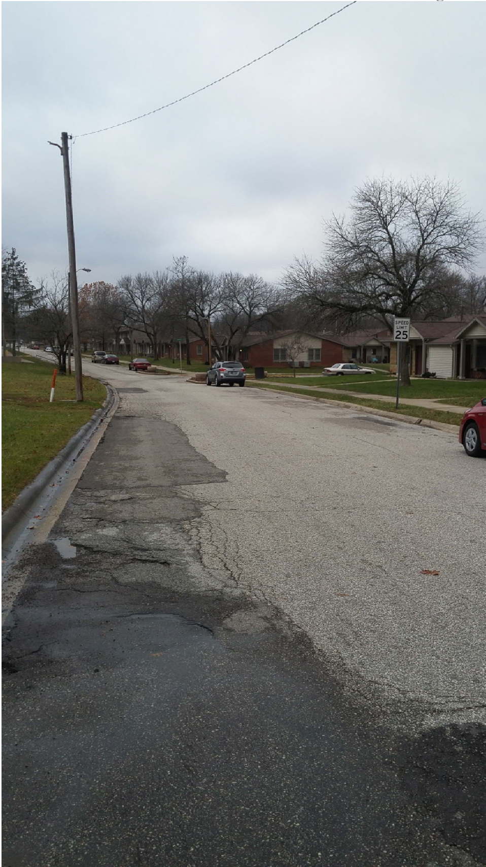
Existing conditions looking west on 12 th Street towards Summit Street
