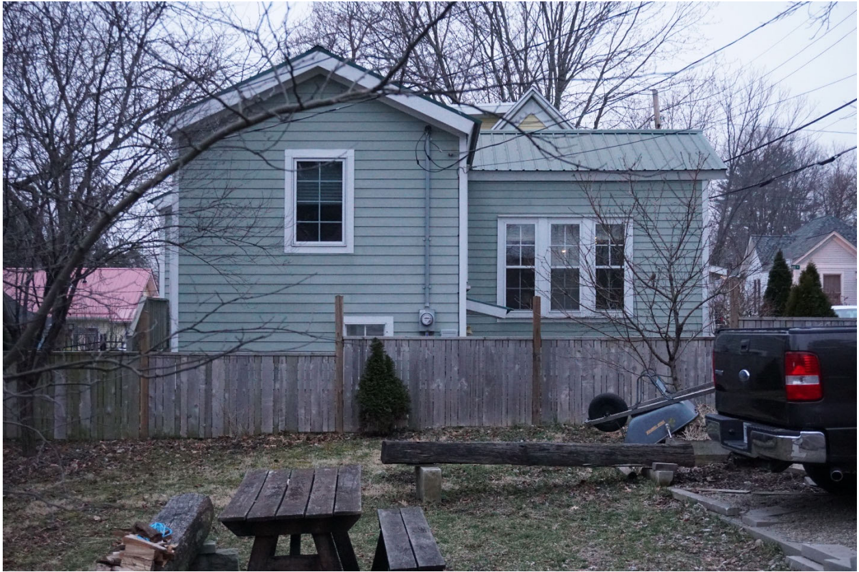
519 W Smith East Elevation View - Looking from ADU/Garage Site
