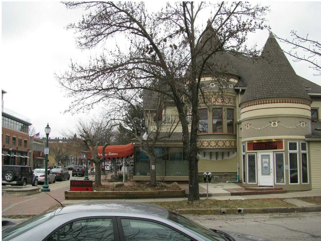
EXISTING EAST ELEVATION PHOTOS
