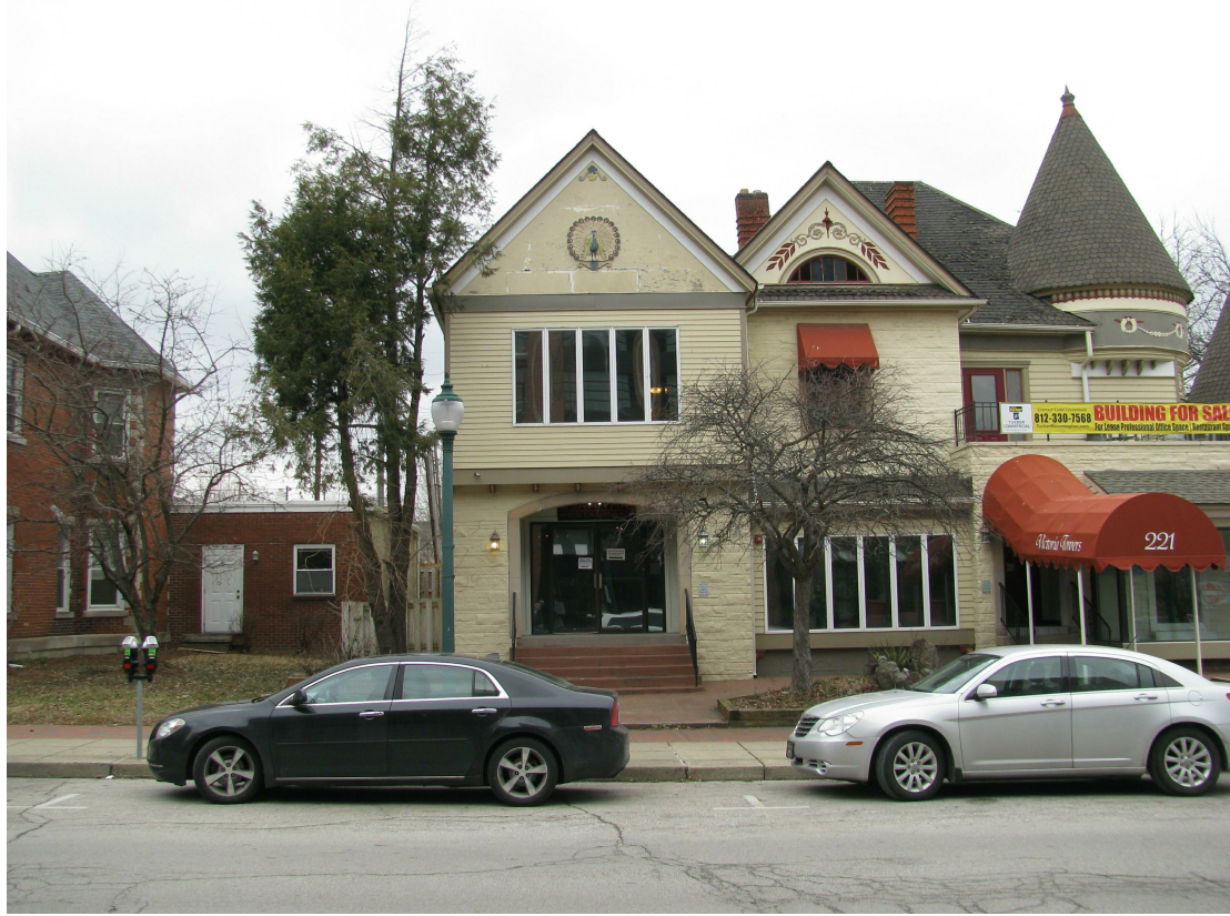
EXISTING SOUTH ELEVATION PHOTOS
