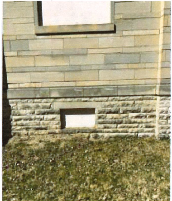
East Façade Basement Window to be Covered
