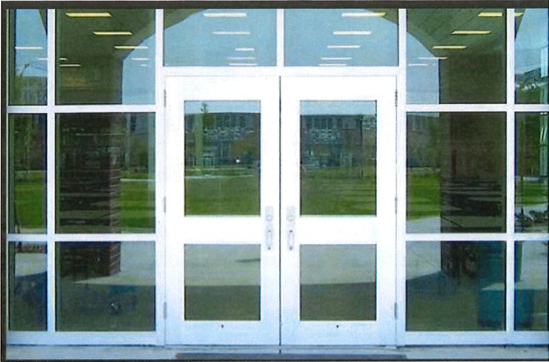
Church Entry Doors (North Façade)
