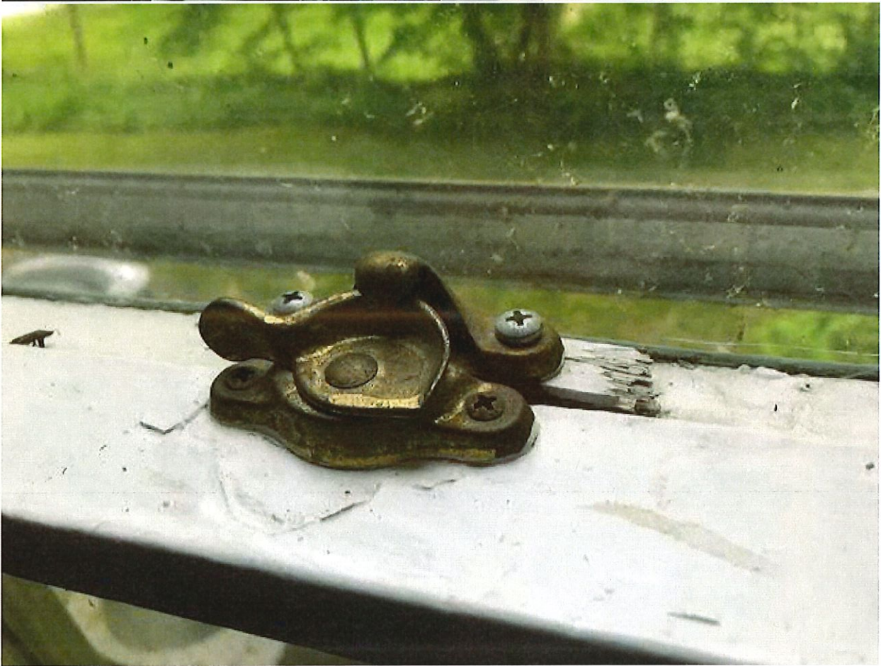
The top picture shows the outside of the window and the incorrectly installed storm window. The middle two pictures show the sash ropes cut and the bottom picture shows the modifications to the window lock.
