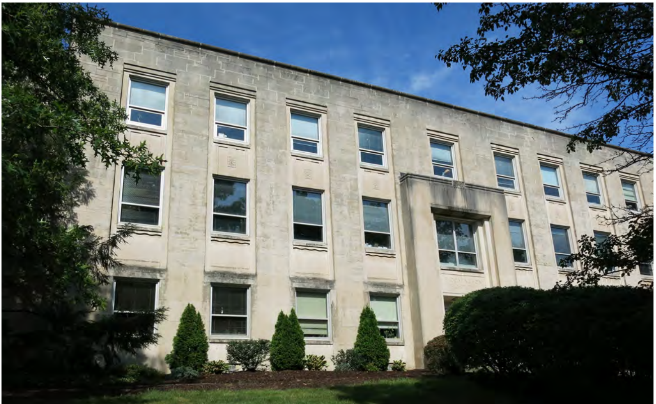
1947 wing, looking northwest, 2018
