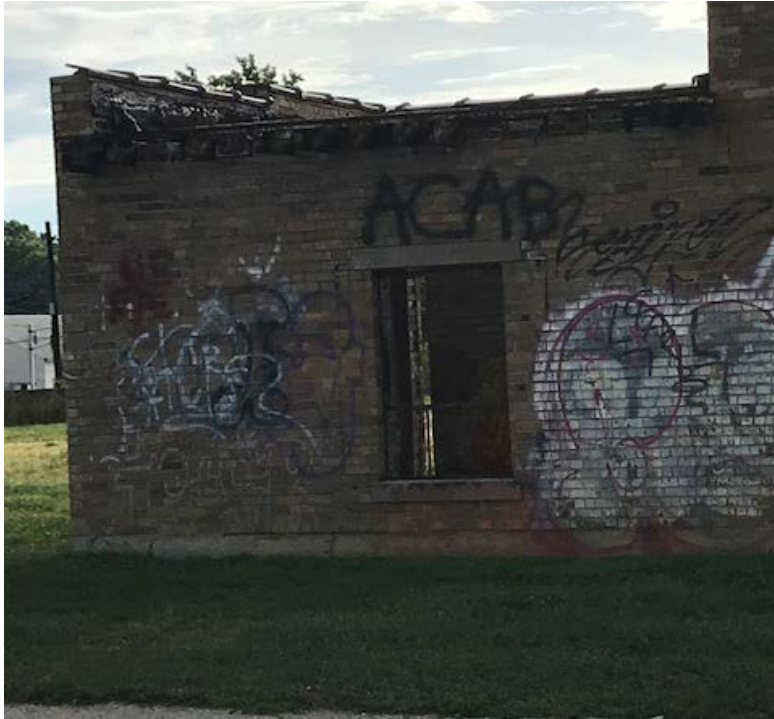
Windows and door on the NW portion of the structure
