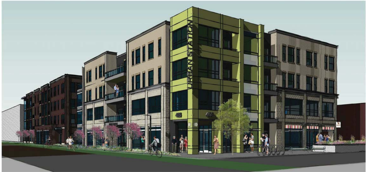
West Bldg. - Northwest Corner
