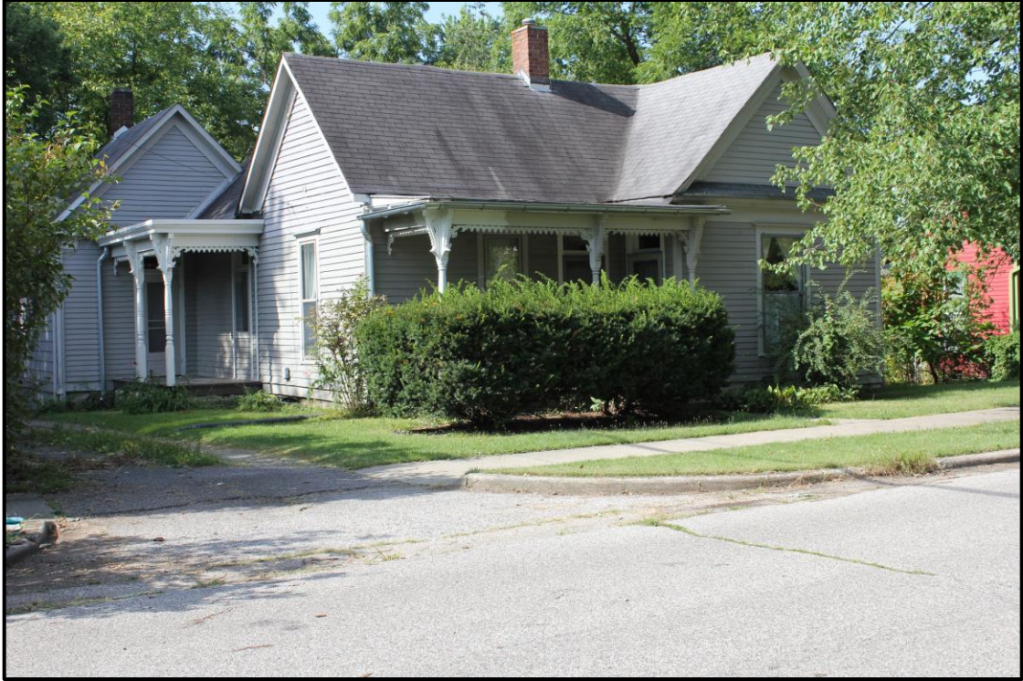
715 W. Eighth Street — Outstanding Architectural Style: Gabled ell with Queen Anne detailing, c. 1895
