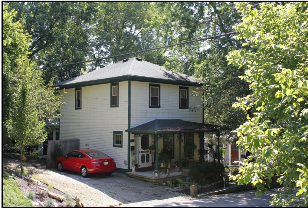
210 N. Elm Street — Contributing Architectural Style: American Foursquare, c. 1920
