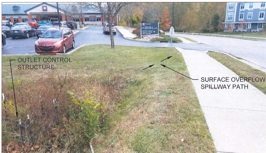
SURFACE OVERFLOW SPILLWAY
