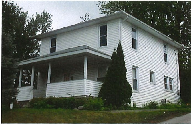
North View of Home from Morton Street/B Line Trail
