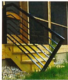
Custom Fabricated Steel Porch Rails and Railing Panels, created locally by Clutch Fabrication
