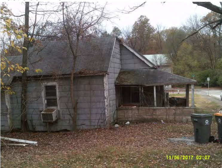
East side looking west- No. 3
