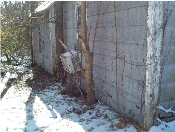
East wall looking south – No. 5
