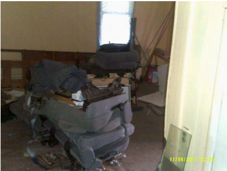
Interior conditions- No. 19
