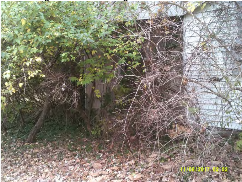
View along east wall - NO 8
