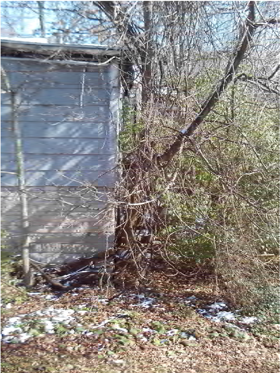
Southwest corner looking east – No. 11
