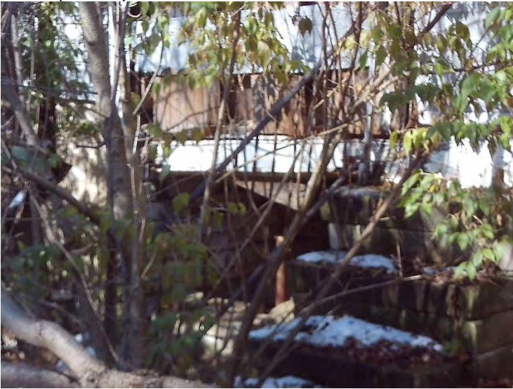
West end of south wall – No. 18
