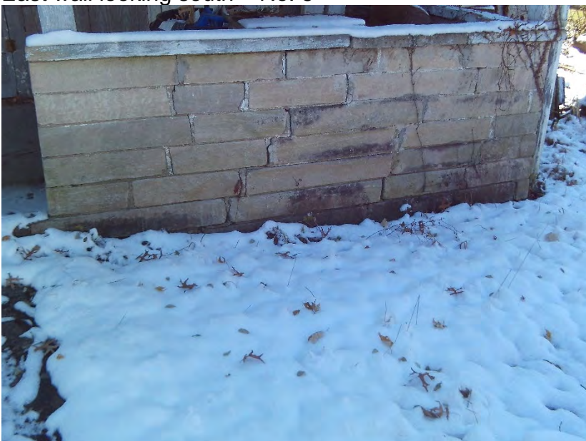
East porch wall - No. 6
