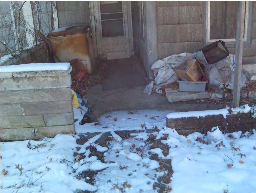
Front porch looking south- No. 19
