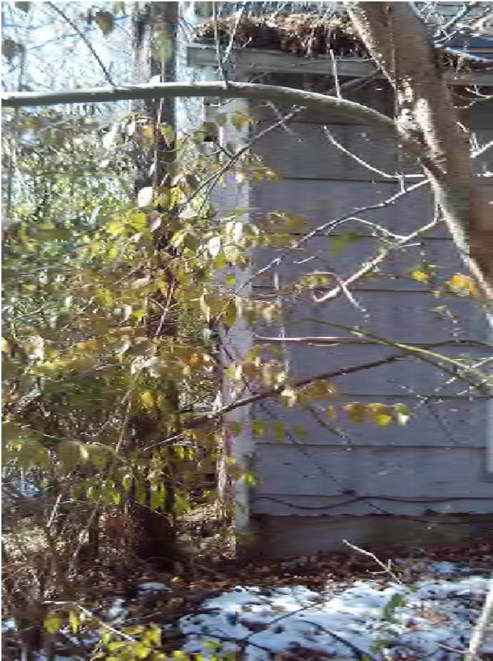
Southeast corner looking west- No. 15
