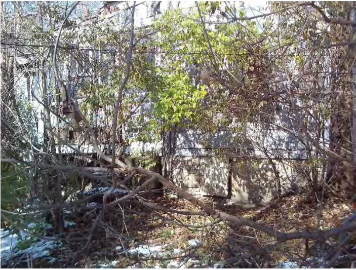
Rear (South) wall – No. 17
