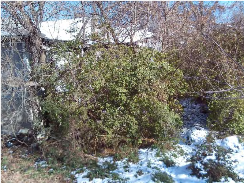
Looking east along south wall - No. 12
