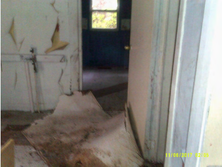
Interior conditions – No. 17
