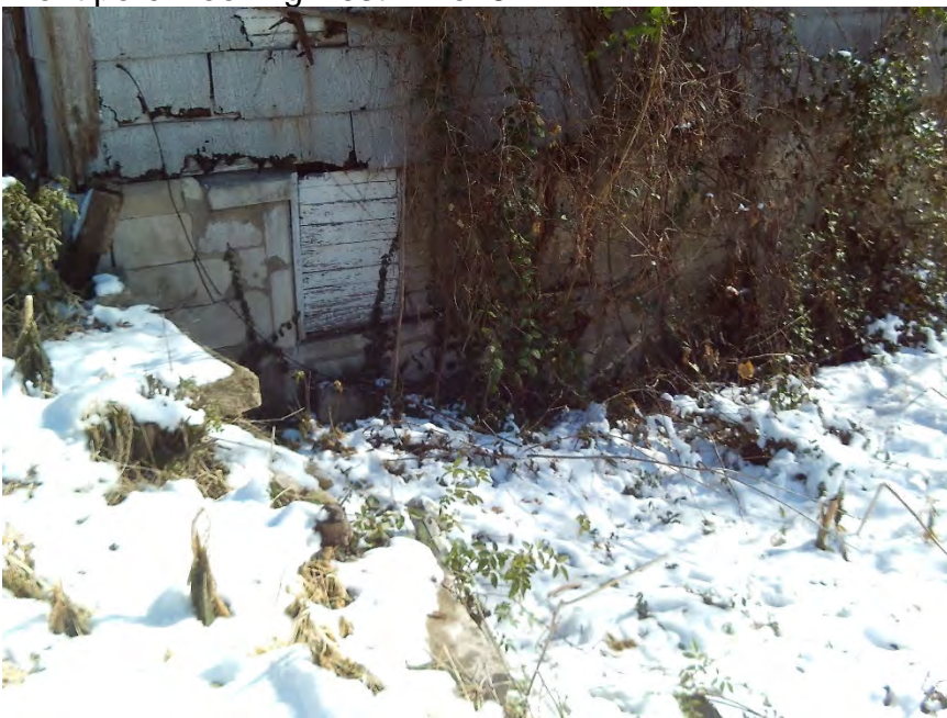
North end of west wall – No. 9
