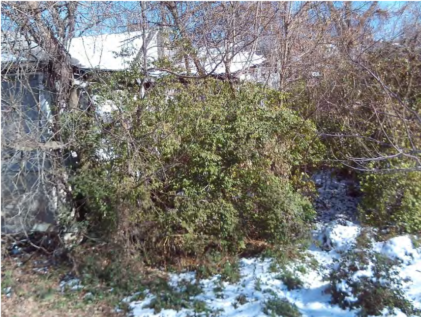
South side looking east - No. 16
