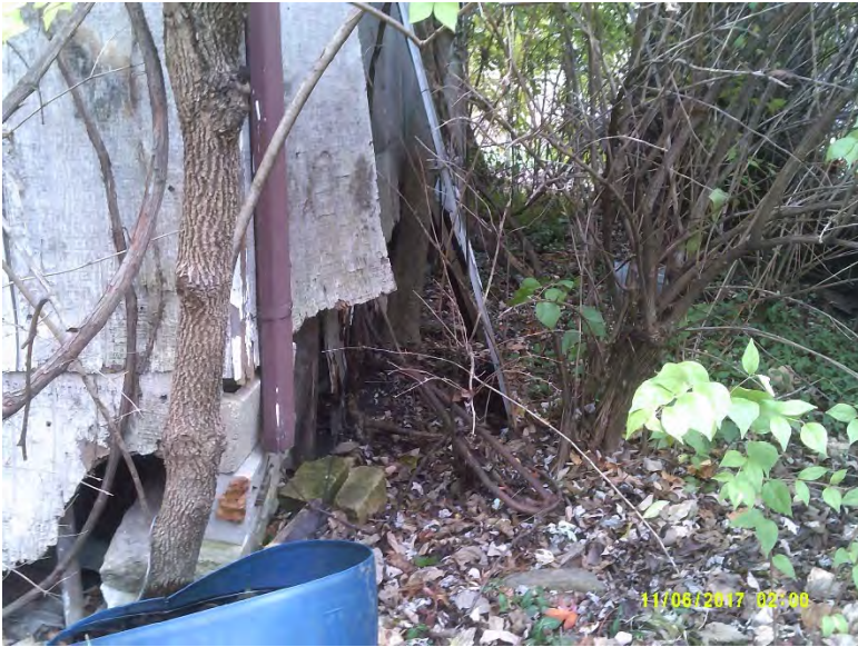
View along south wall – Large tree next to house No. 7
