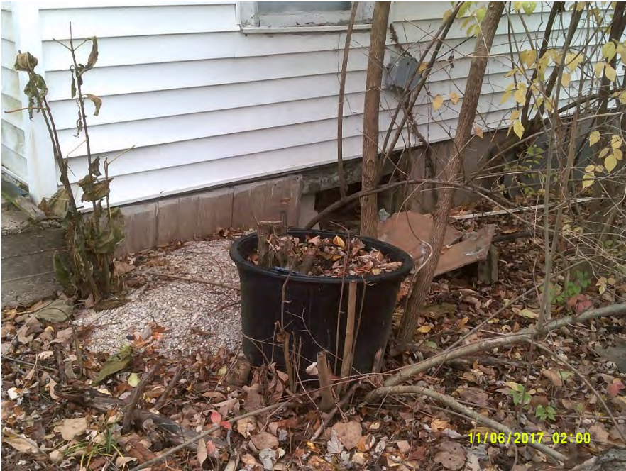
Uncovered crawl space access on west side- No 4
