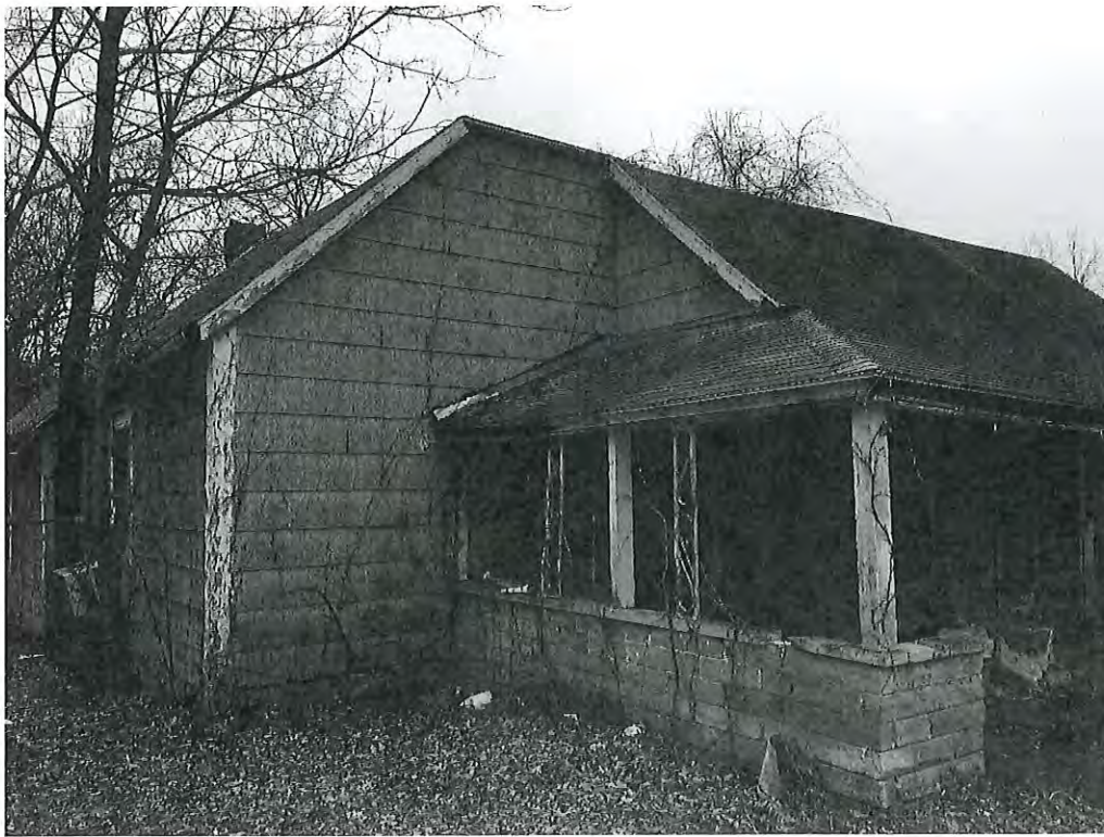
Front Porch Detail
