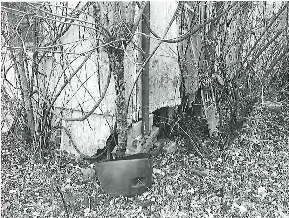
Rear Foundation/Floor Conditions
