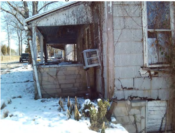
Front porch looking west – No. 8
