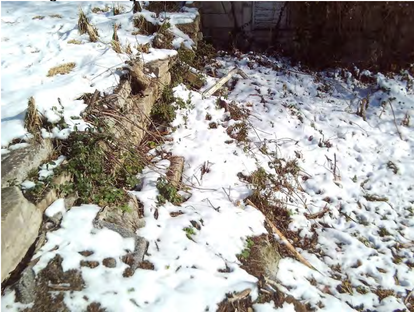
Looking east at northwest retaining wall – No. 13
