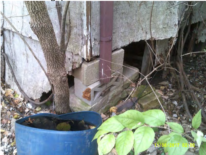
Foundation at southwest corner No. 6
