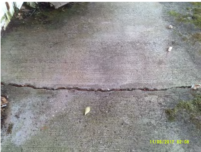
Front porch conditions – No. 21
