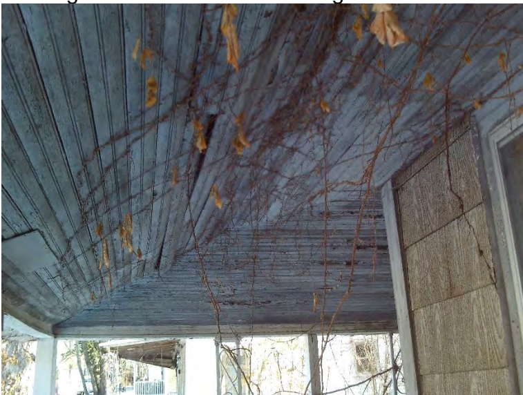
Front porch roof – No. 14
