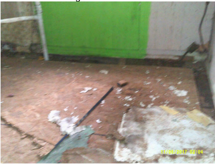
Interior conditions – No. 14
