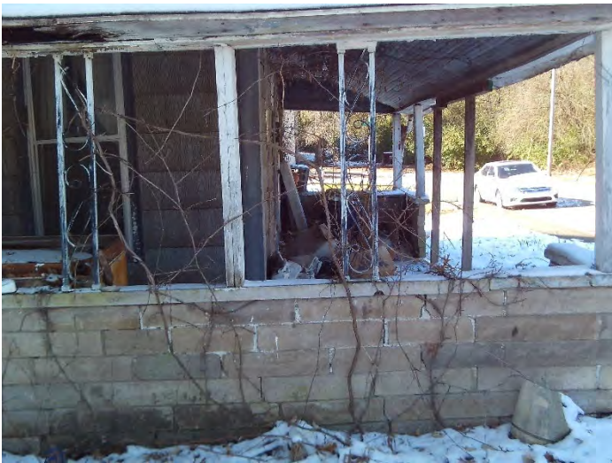
Front porch looking east – No. 7
