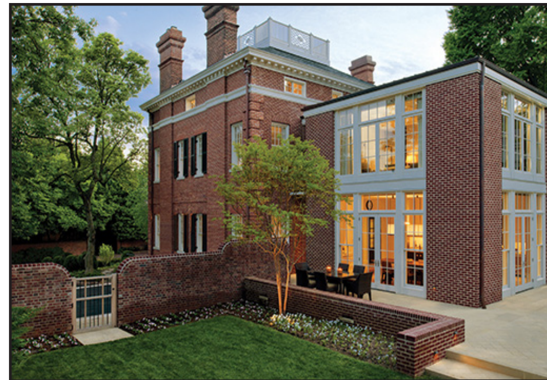
This glass and brick structure is a harmonious addition set back and connected to the rear of the Colonial Revival-style brick house. The addition is Compatible in materials, color, and proportion. It is Differentiated in that it is subordinate to the historic building and does not unify the two volumes into a single architectural whole. Photograph courtesy of the Secretary of the Interior's Preservation Brief # 14.
