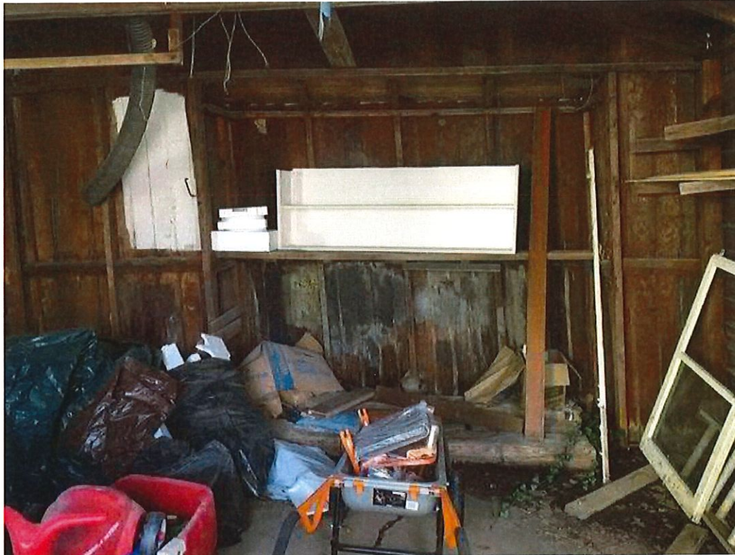
Looking toward back of garage interior
