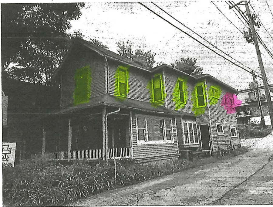
Front view of subject, looking southeast
