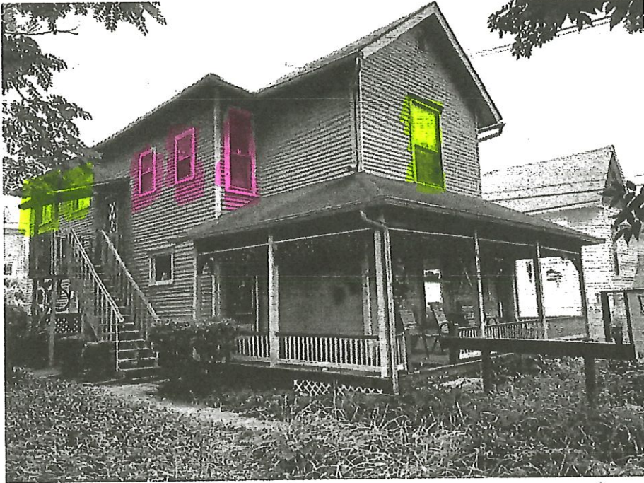
Front view of subject, looking southwest
