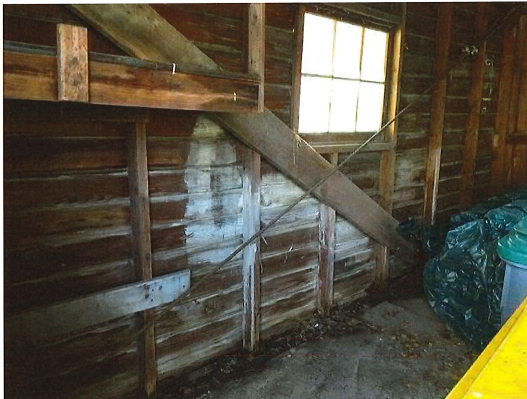
Looking at interior of east wall
