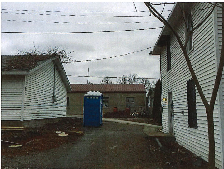
Space between existing House and Garage where proposed addition is planned to be built.
