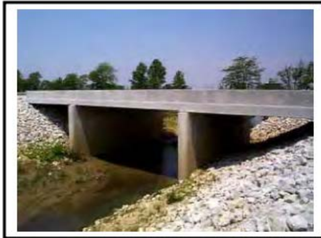
Figure 1:6-4: Continuous Reinforced Concrete Slab Bridge
