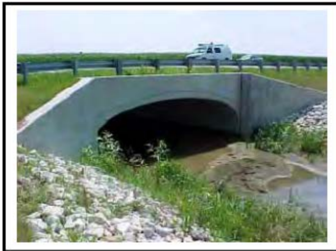
Figure 1:6-5: Precast Concrete Underfill Bridge
