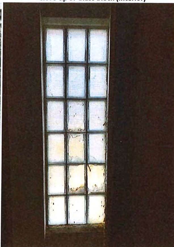
Close-up of Glass Block (Interior)
