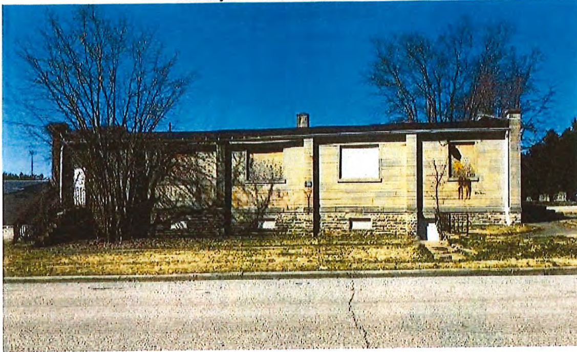
East Façade – From Walker Street
