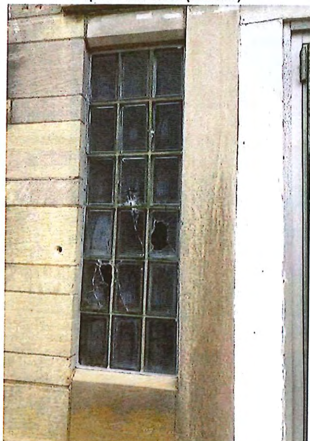
Close-up of Glass Block (Exterior)
