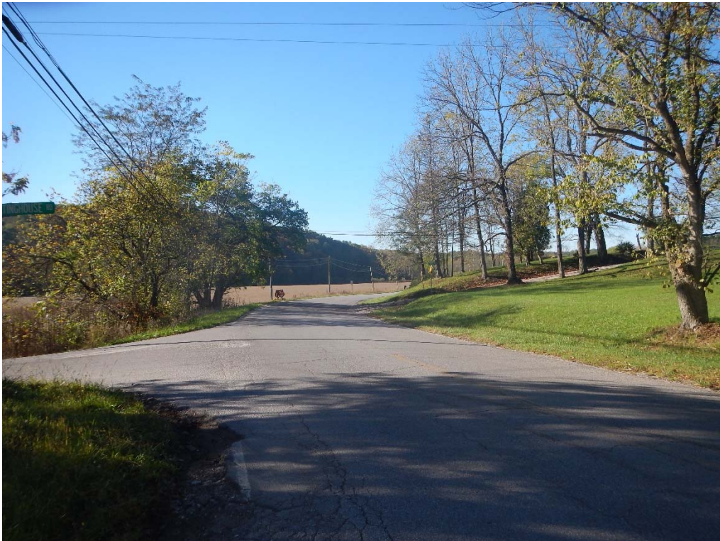
Photo 2. Facing south along Old SR 37 toward the intersection of Boltinghouse Rd.
