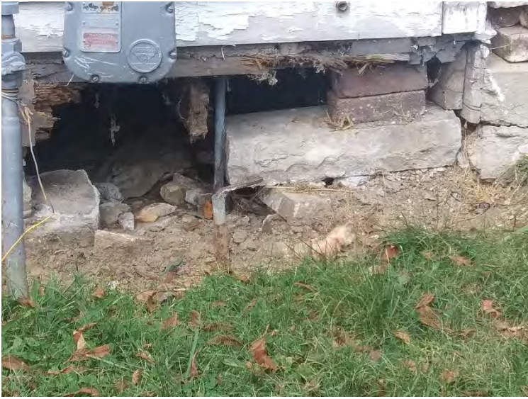
Southeast corner of foundation wall
