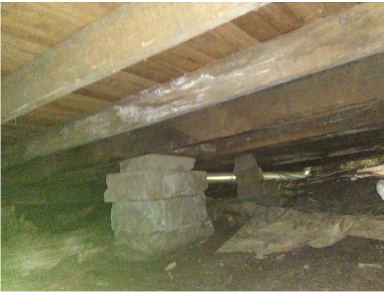
South part of crawl space
