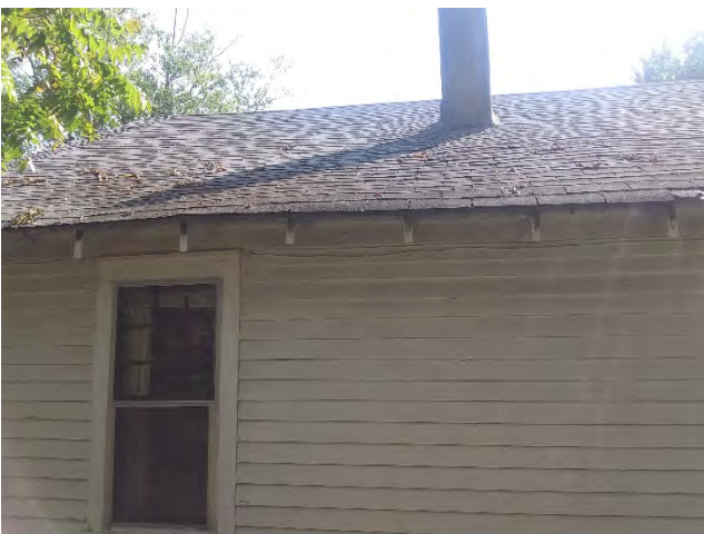
Wavy roof on north side
