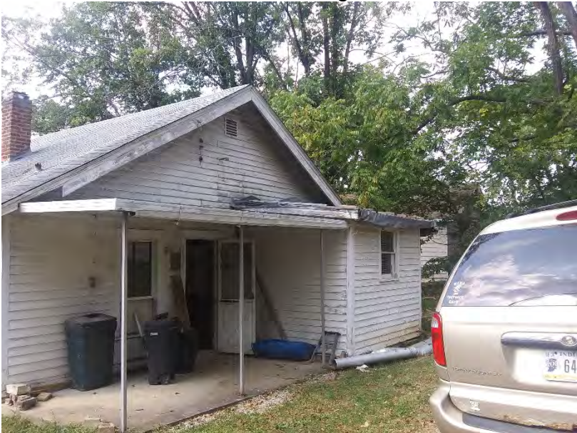
East side porch roof and bathroom addition
