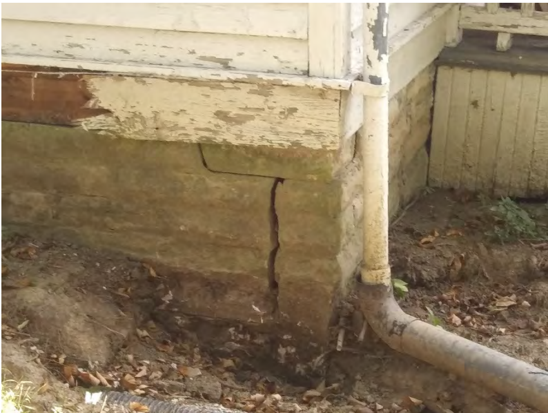
Foundation at Northwest corner
