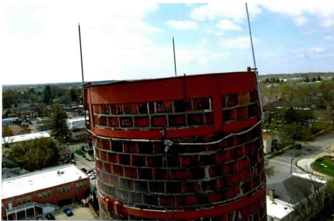
Photo 2. Good condition of the encircling plate and connections to the upper band. Note the slope ( \pm 4^\circ ) of the top of the chimney due to the lean toward the southeast direction.
