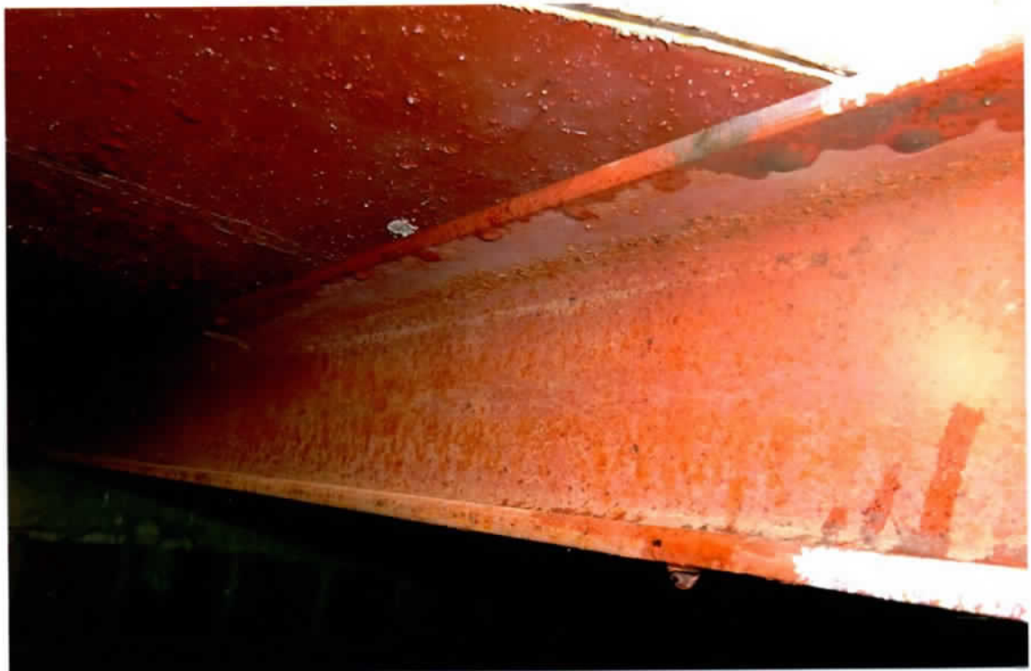
Photo 4. Good condition of the roof plate underside and 4" deep support beam (near center of roof).
