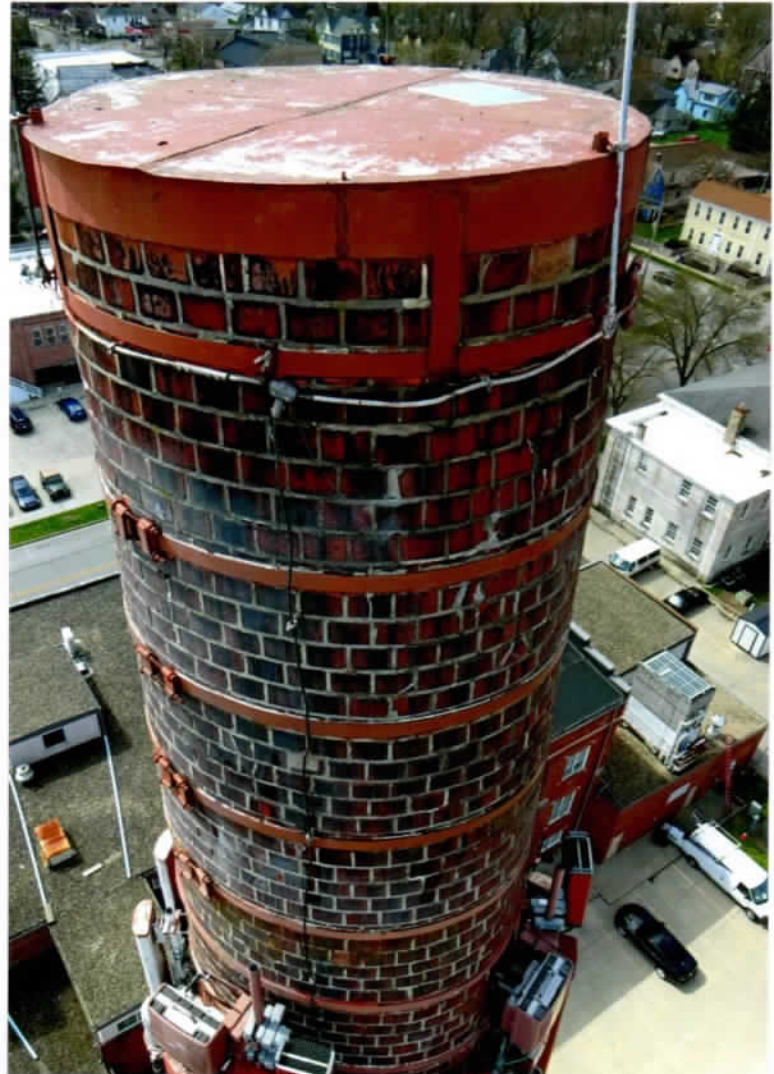
Photo 15. Overall good exterior condition of the upper elevations of the northeast side. Mortar joints appeared repointed within the past 15 years. LPS cables, bands and roof were secure.
