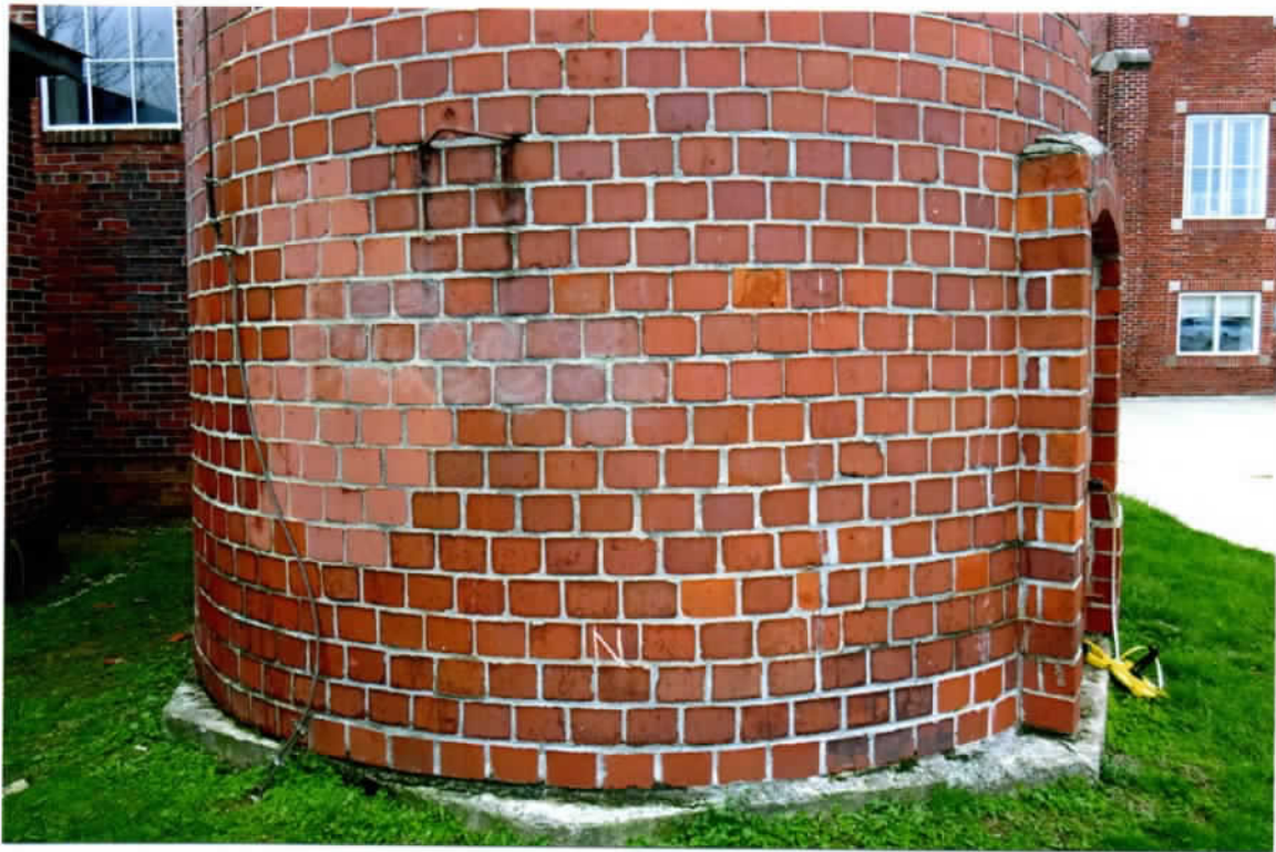
Photo 59. Good exterior condition of the lower north side at grade. The concrete foundation below the brick chimney was slightly eroded.
