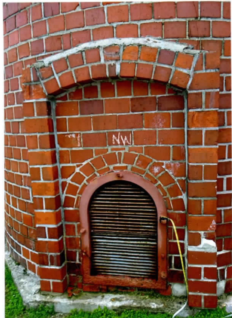
Photo 65. Close-up of the brick chimney not bearing on the concrete foundation (east side). No concerns were seen with the concrete directly below the brick wall in this region.
