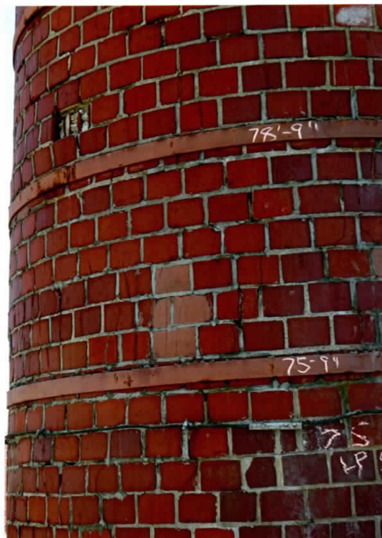
Photo 37. Local area of bulged and spalled bricks (80' level, northwest side). Several brick faces were partially dislodged.
