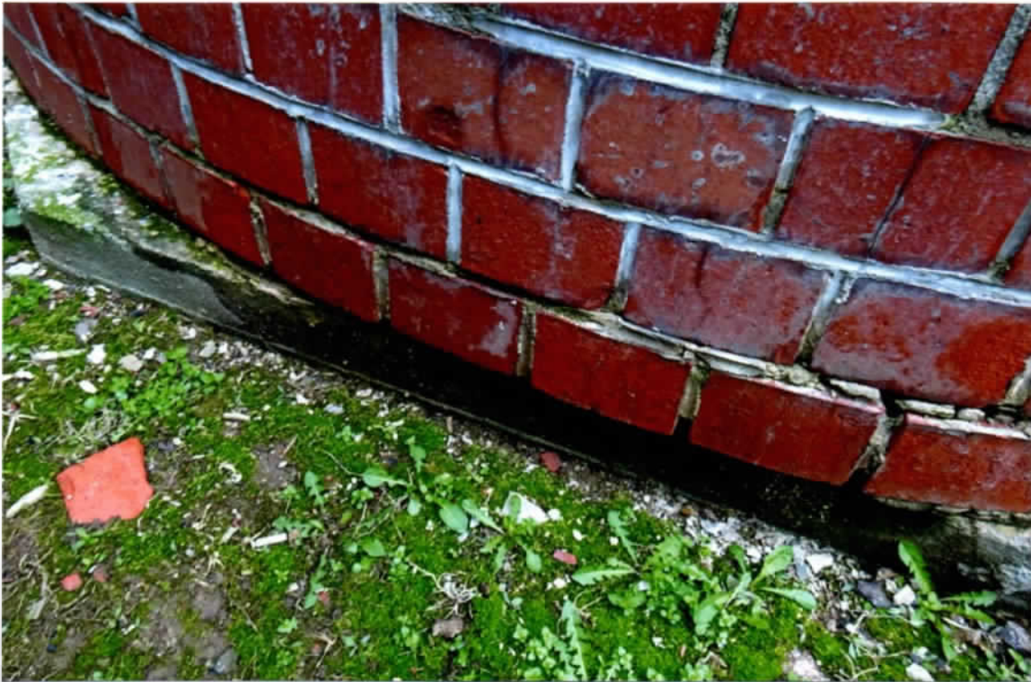
Photo 65. Close-up of the brick chimney not bearing on the concrete foundation (east side). No concerns were seen with the concrete directly below the brick wall in this region.
