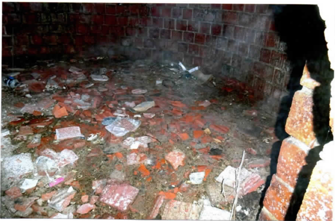
Photo 70. Approximately 8" of debris and brick faces in the chimney base near grade (south side). Note the numerous brick faces in the debris.
