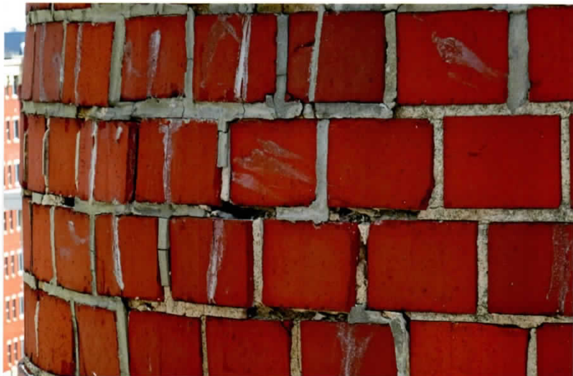
Photo 32. Close-up of the bulged region with eroded joints (101' level, northwest side).
