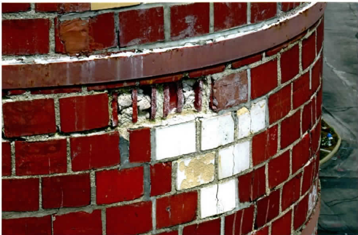
Photo 36. Close-up of the spalled brick faces and eroded mortar joints in the course below the 81'-10" level band, southwest side.
