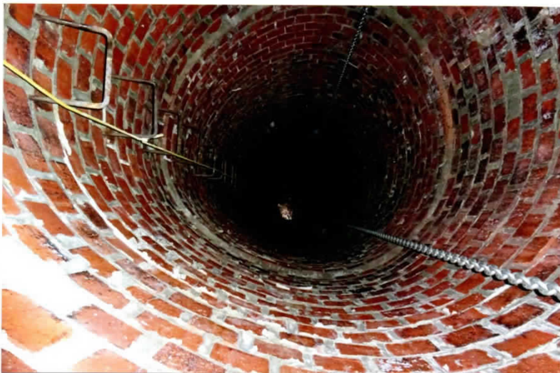
Photo 11. Good interior condition of the upper elevations looking down from the roof. Mortar joints in the uppermost \pm 15' appeared to have been repointed.
