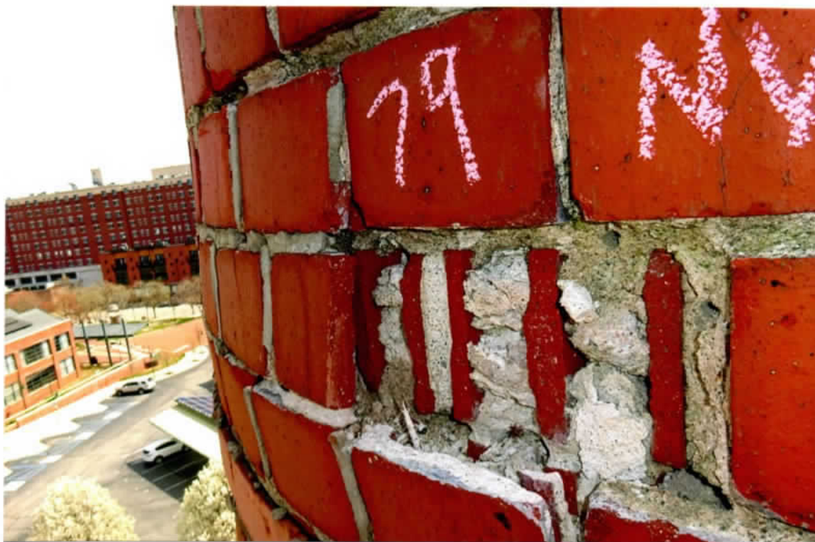
Photo 39. Close-up of the spalled and partially dislodged brick faces near the 80' level, northwest side.
