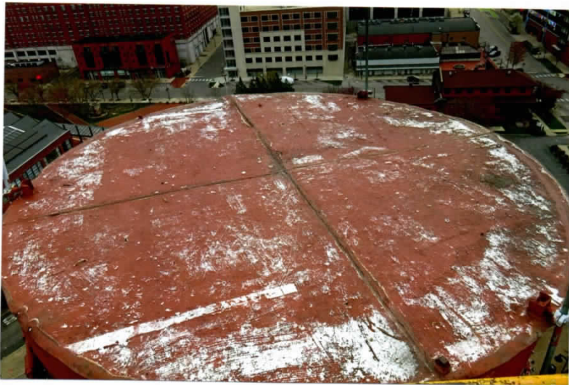
Photo 17. Good condition of the roof plate (looking from west side). Note only the weathered paint. The roof plate and support beams on the underside were secure.
