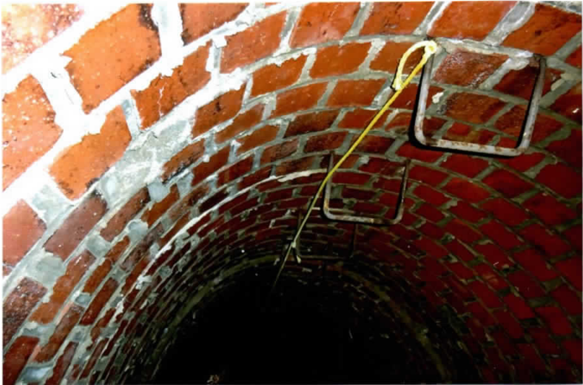
Photo 9. Good interior condition of the upper elevations looking down from the roof (north side). Mortar joints in the uppermost \pm 15' appeared to have been repointed.
