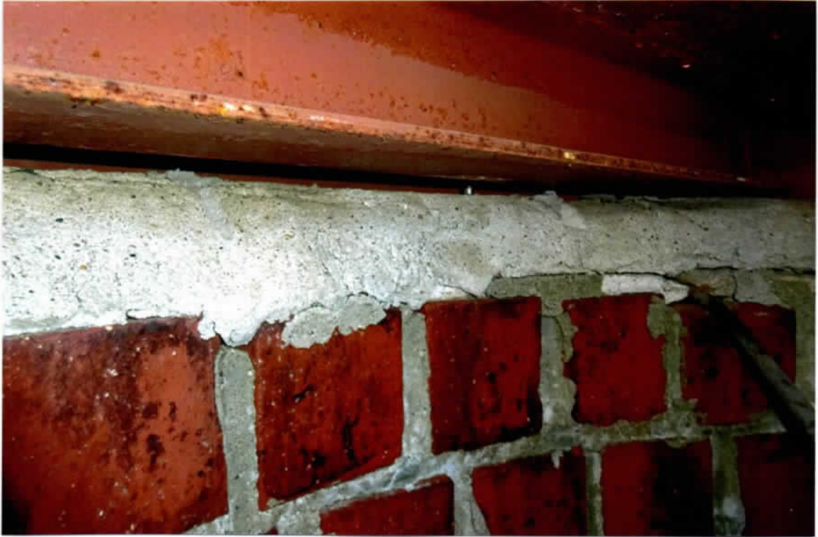
Photo 5. Good interior condition of the cap, brick faces and mortar joints (upper courses of north side). Mortar joints in the upper elevations appeared repointed. No concerns were identified.
