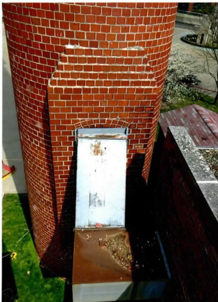
Photo 55. Good condition of the corbelled courses above the extended wall surrounding the original breeching duct opening (south side between the 30' and 20' levels).
