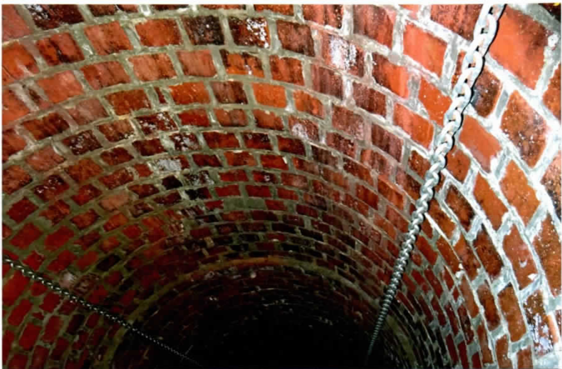
Photo 10. Good interior condition of the upper elevations looking down from the roof (south side). Mortar joints in the uppermost \pm 15' appeared to have been repointed.
