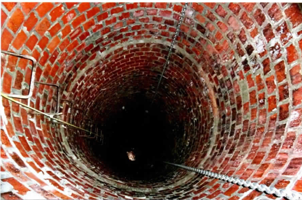
Photo 12. Good interior condition local to the 132' level shelf (wall thickness change). Mortar joints below the 125' level were in fair condition as open and cracked joints were identified.
