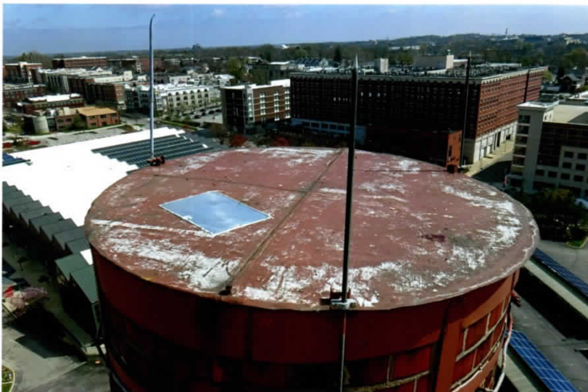
Photo 1. Good condition of the steel roof atop the chimney. Note only the weathered paint. The patch plate was recently installed.
