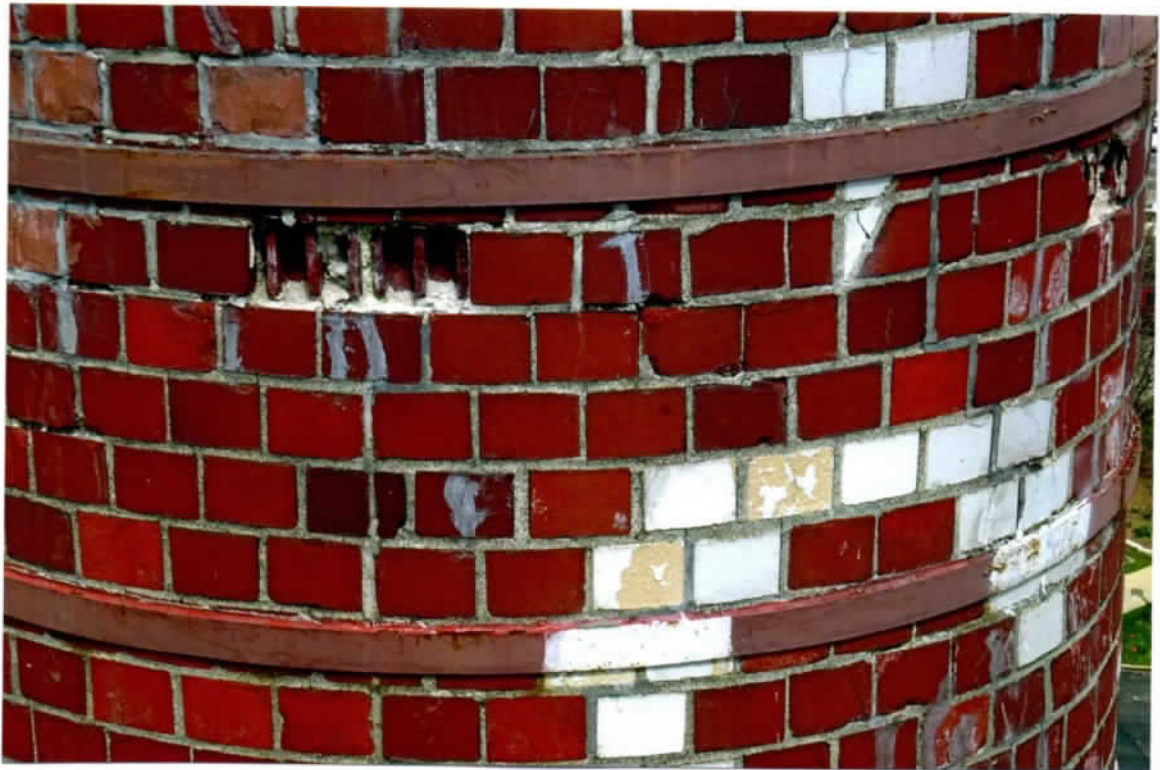
Photo 35. Close-up of the spalled brick faces in the course below the 89'-8" level band, south side.
