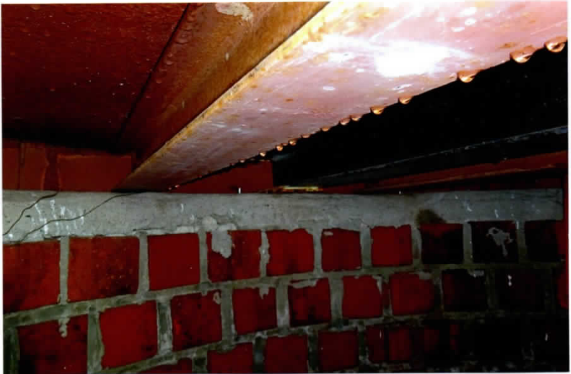
Photo 7. Good interior condition of the cap, brick faces and mortar joints (upper courses of east side). Note the good condition of the \pm 3 " cement cap atop the brick wall.
