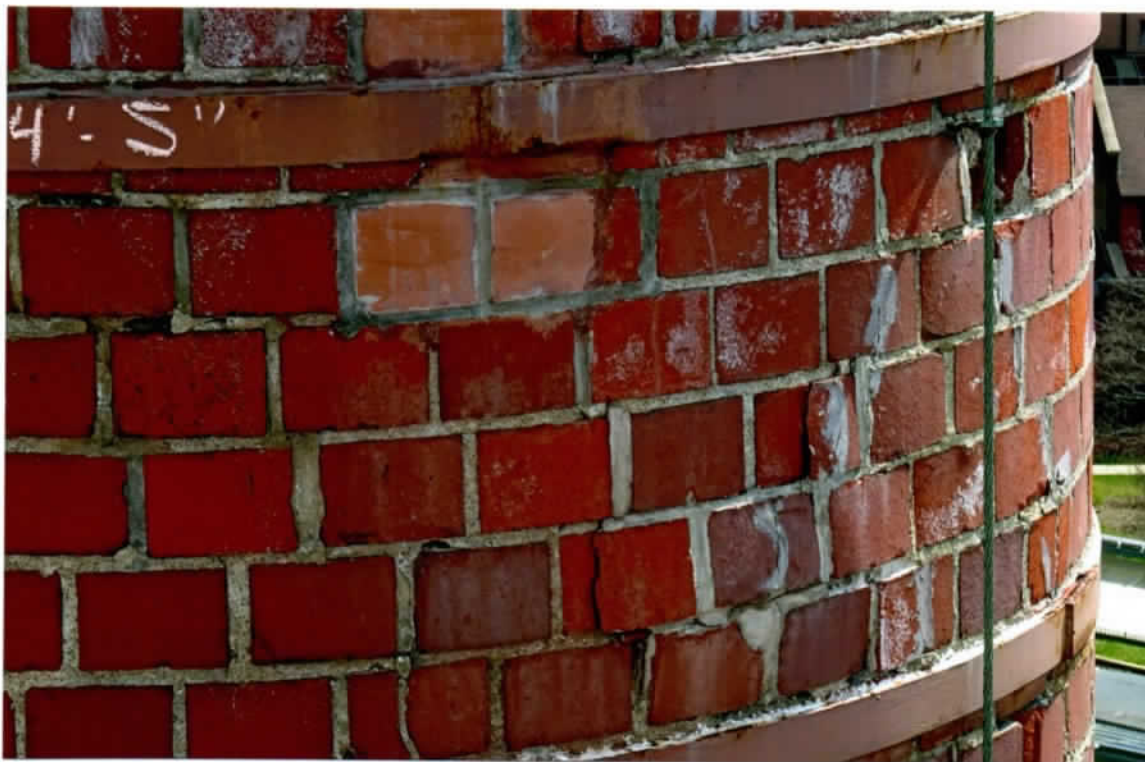
Photo 30. Local area of cracked and spalled brick faces (83' level, southwest side). Note the past repairs to replace several bricks near the upper band.
