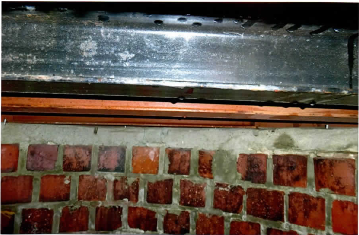
Photo 6. Good interior condition of the cap, brick faces and mortar joints (upper courses of south side). Note the good condition of the \pm 3" cement cap atop the brick wall.
