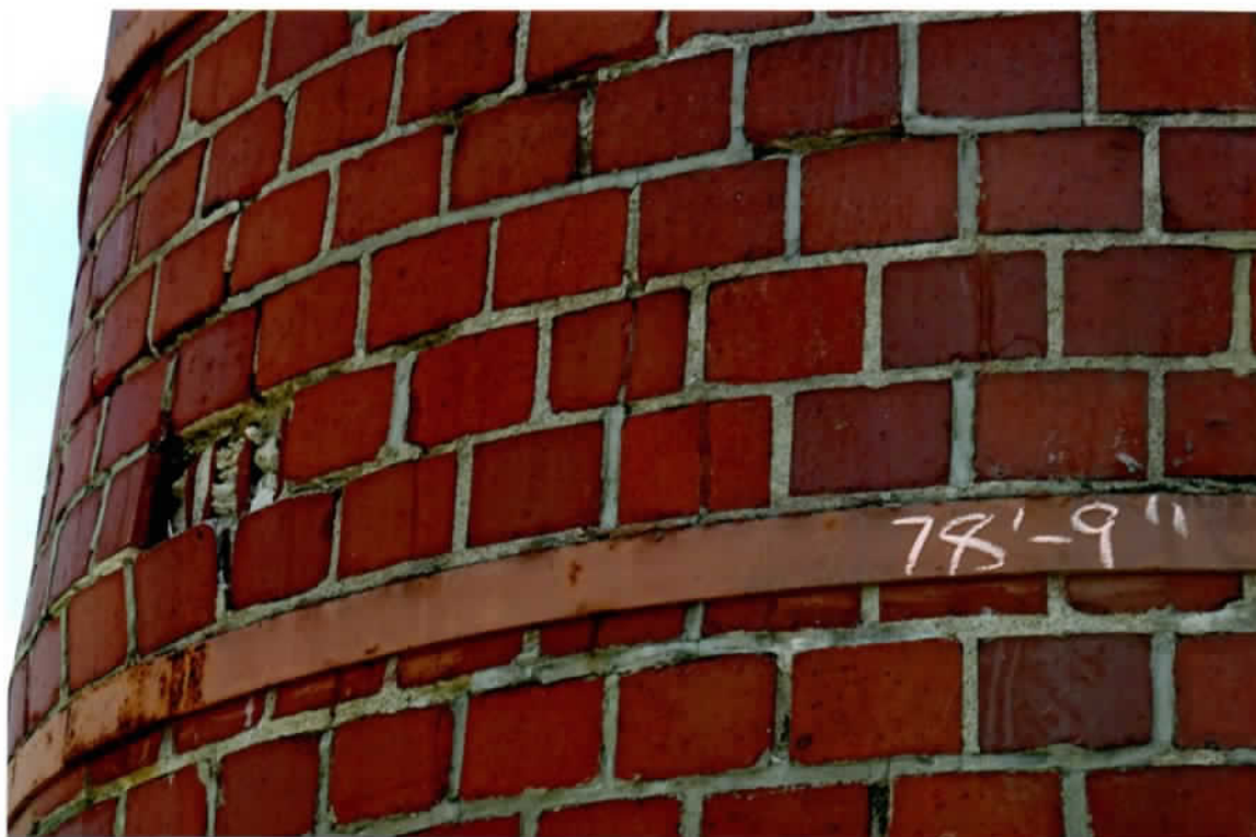
Photo 37. Local area of bulged and spalled bricks (80' level, northwest side). Several brick faces were partially dislodged.
