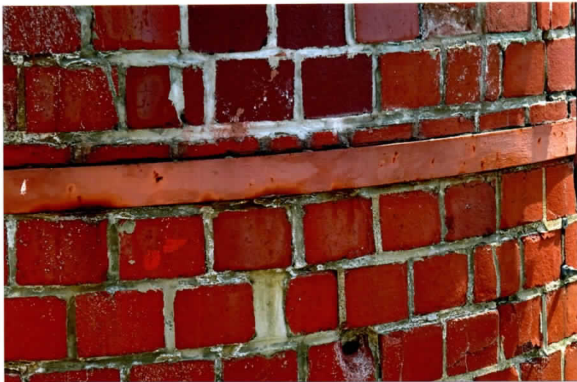
Photo 53. Close-up of the spalled brick face below the 41'-11" level band, west side.
