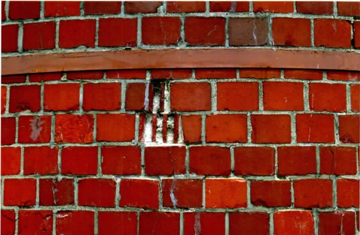
Photo 44. Close-up of the spalled brick faces below the 57'-7" level band, south side.
