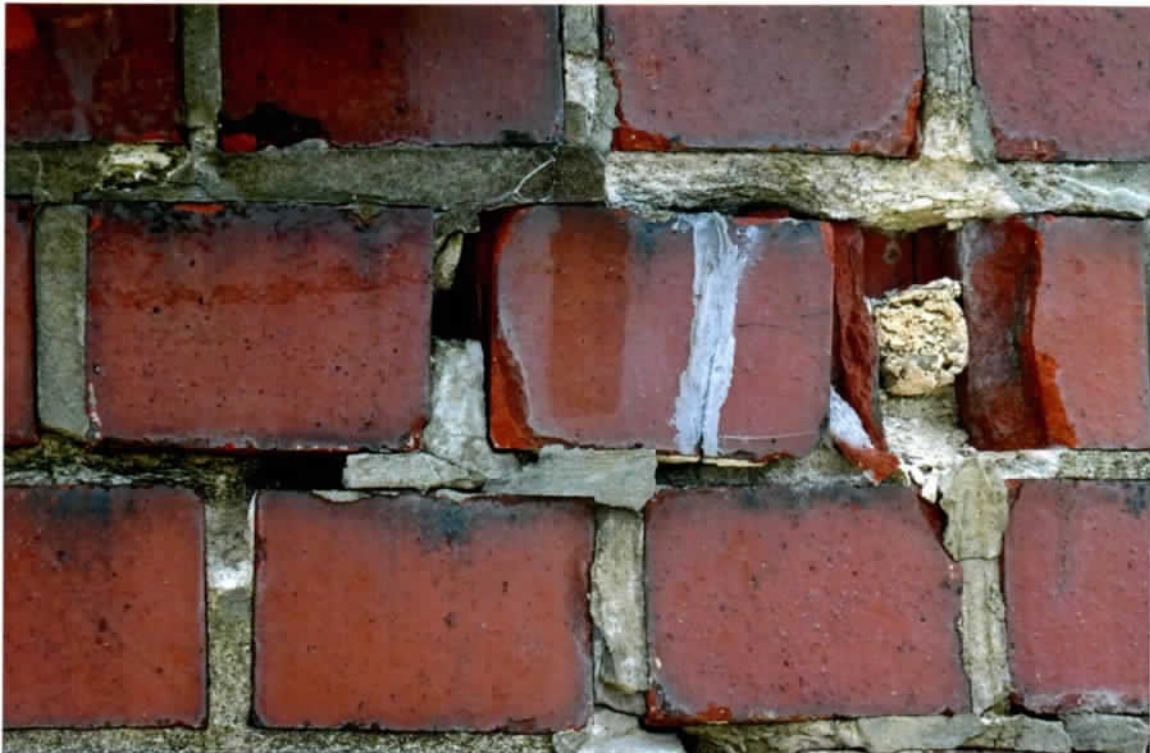
Photo 20. Close-up of the cracked and spalled bricks and dislodged mortar (130' level, west side).
