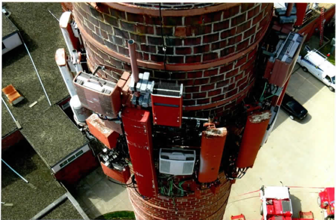
Photo 24. Good condition of the existing antennas and RRF units (northeast side). Nearly all components were supported by three exterior bands (123'-6", 121'-6" and 118'-4" levels).
