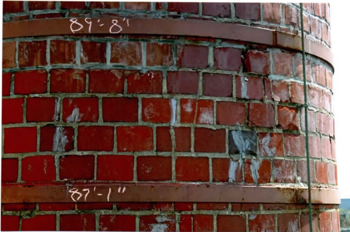
Photo 29. Local area of cracked and spalled brick faces (89' level, southwest side). Numerous generations of repointing work were identified in this region.
