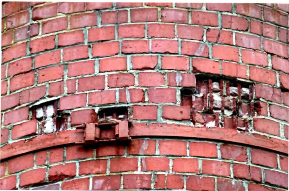
Photo 46. Close-up of the spalled brick faces above the 41'-11" level band, south side.
