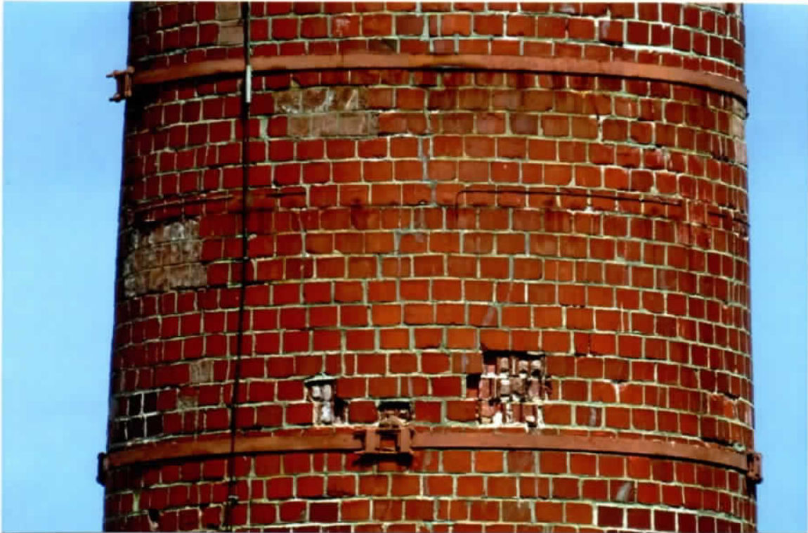
Photo 45. Poor exterior condition of the south side between the 49' and 41' levels. Note the numerous spalled and eroded brick faces.
