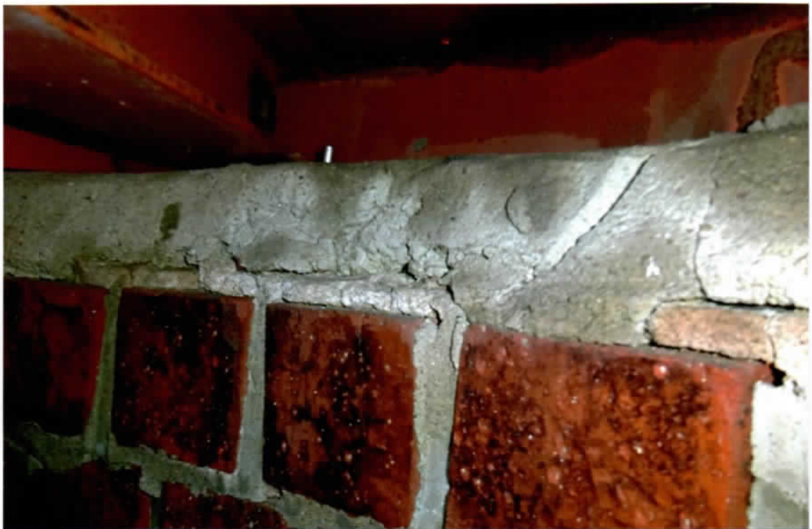
Photo 8. Good interior condition of the cap, brick faces and mortar joints (upper courses of west side). Note the good condition of the \pm 3 " cement cap atop the brick wall.
