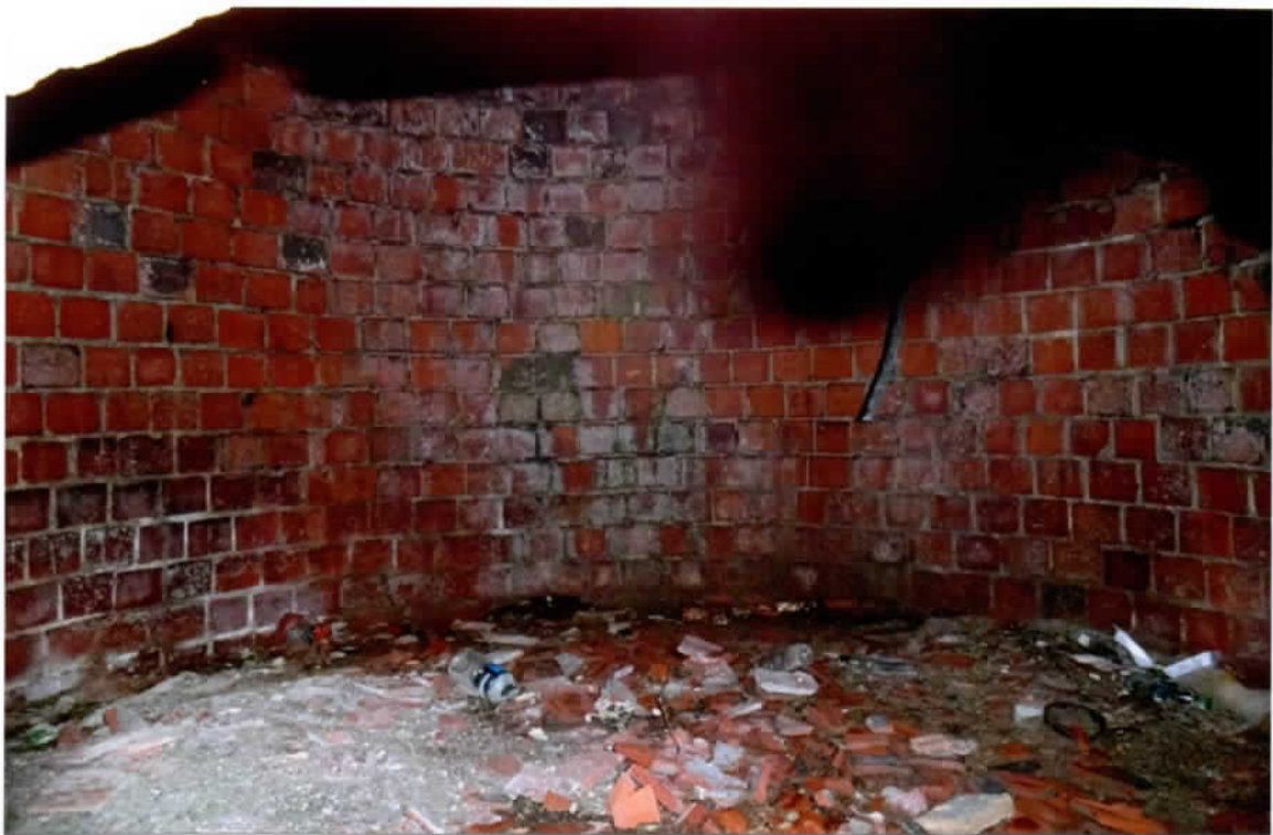
Photo 68. Fair interior condition of the lower brick wall (east and southeast sides). No immediate concerns were seen throughout the lower elevations of the outer wall.
