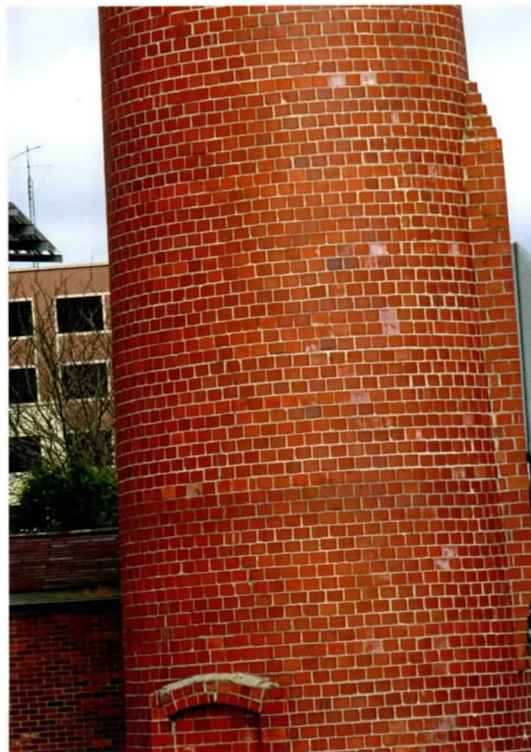
Photo 53. Close-up of the spalled brick face below the 41'-11" level band, west side.
