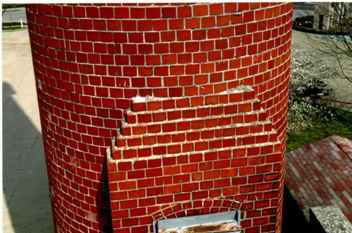
Photo 55. Good condition of the corbelled courses above the extended wall surrounding the original breeching duct opening (south side between the 30' and 20' levels).
