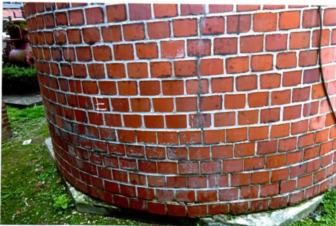
Photo 61. Good exterior condition of the lower east side at grade. The brick chimney overhung the concrete foundation by several inches in this region.
