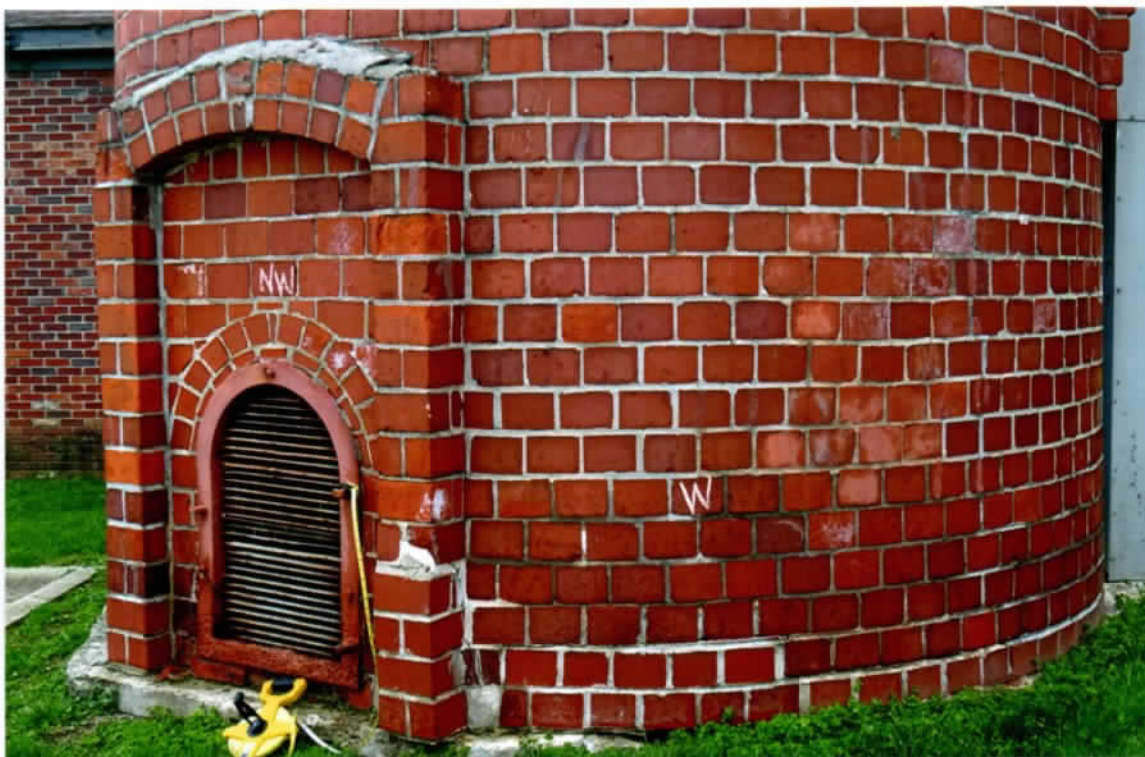
Photo 62. Good exterior condition of the lower west side at grade. The concrete foundation below the brick chimney was slightly eroded.
