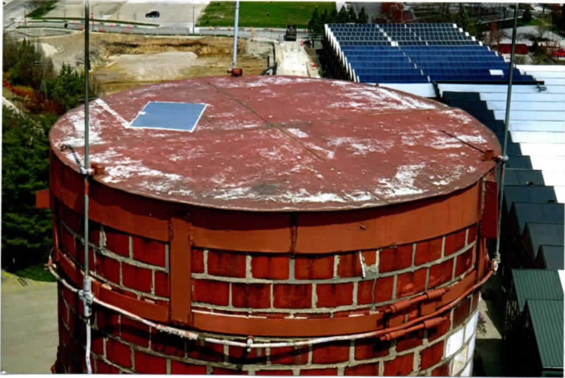
Photo 13. Overall good exterior condition of the upper elevations of the south side. Mortar joints appeared repointed within the past 15 years. LPS cables, bands and roof were secure.
