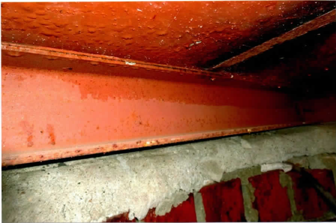
Photo 3. Good condition of the roof plate underside and 4" deep support beam (north side). Also note the good condition of the 3" thick cement cap atop the uppermost course.
