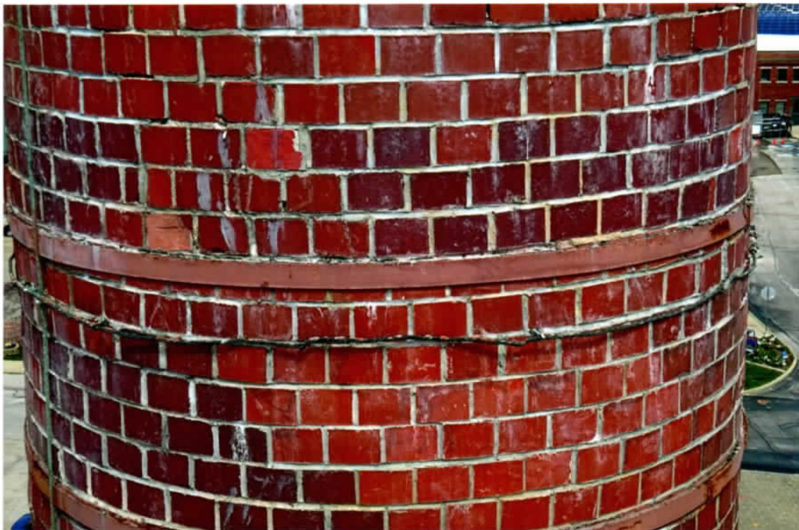
Photo 41. Fair exterior chimney of the south side between the 78' and 73' levels. No spalled bricks existed in this region. All LPS cables were secure.
