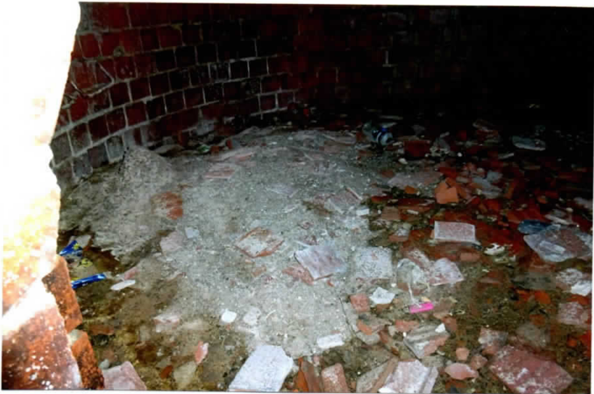
Photo 69. Approximately 8" of debris and brick faces in the chimney base near grade (north side). Note the numerous brick faces in the debris.
