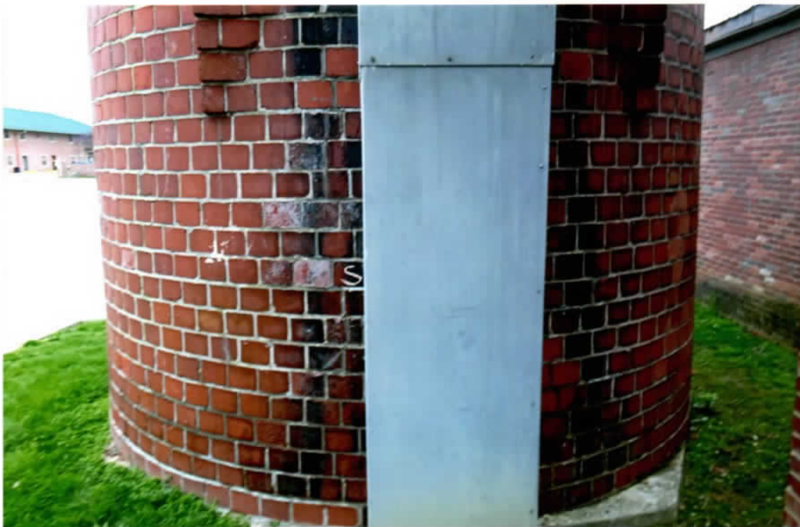
Photo 60. Good exterior condition of the lower south side at grade. Note only staining on the brick chimney from past leakage at the duct sill.
