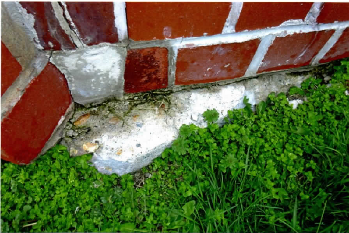
Photo 63. Close-up of the eroded concrete along the top of the foundation (west side).
