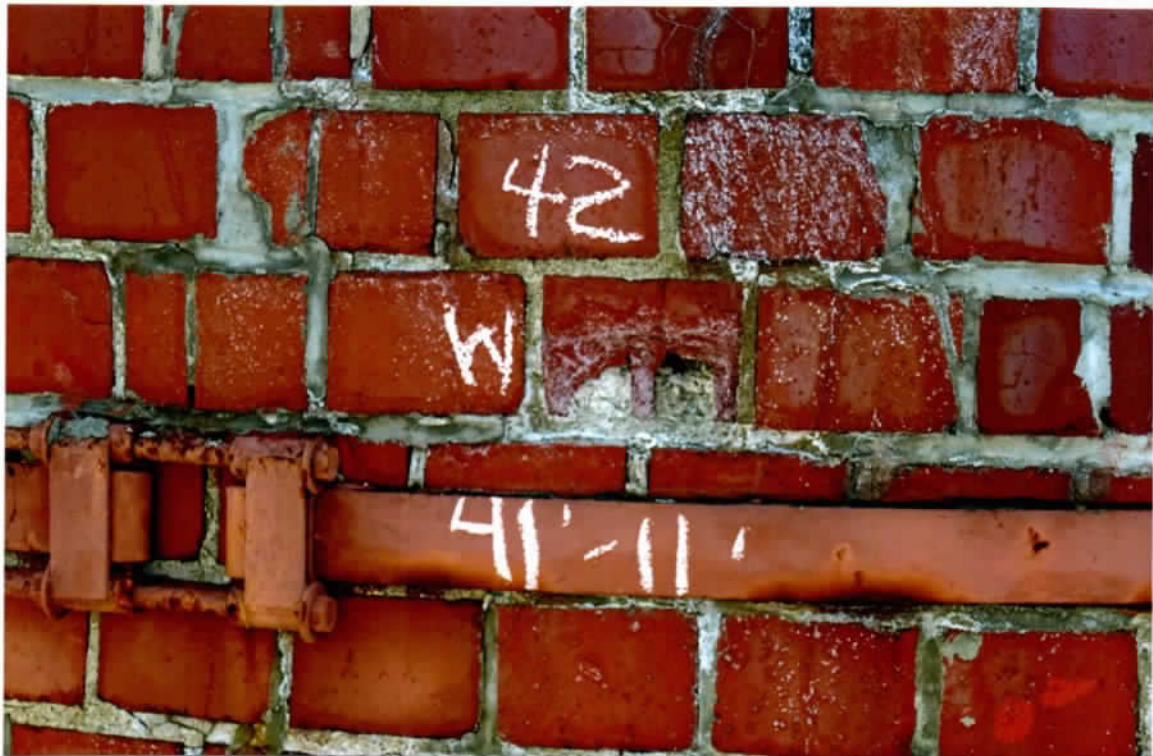
Photo 52. Close-up of the spalled brick face above the 41'-11" level band, west side.
