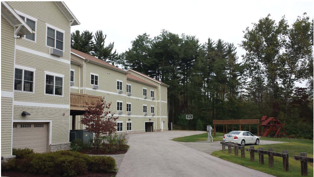
East side of building, facing north. Existing deck to be removed.
