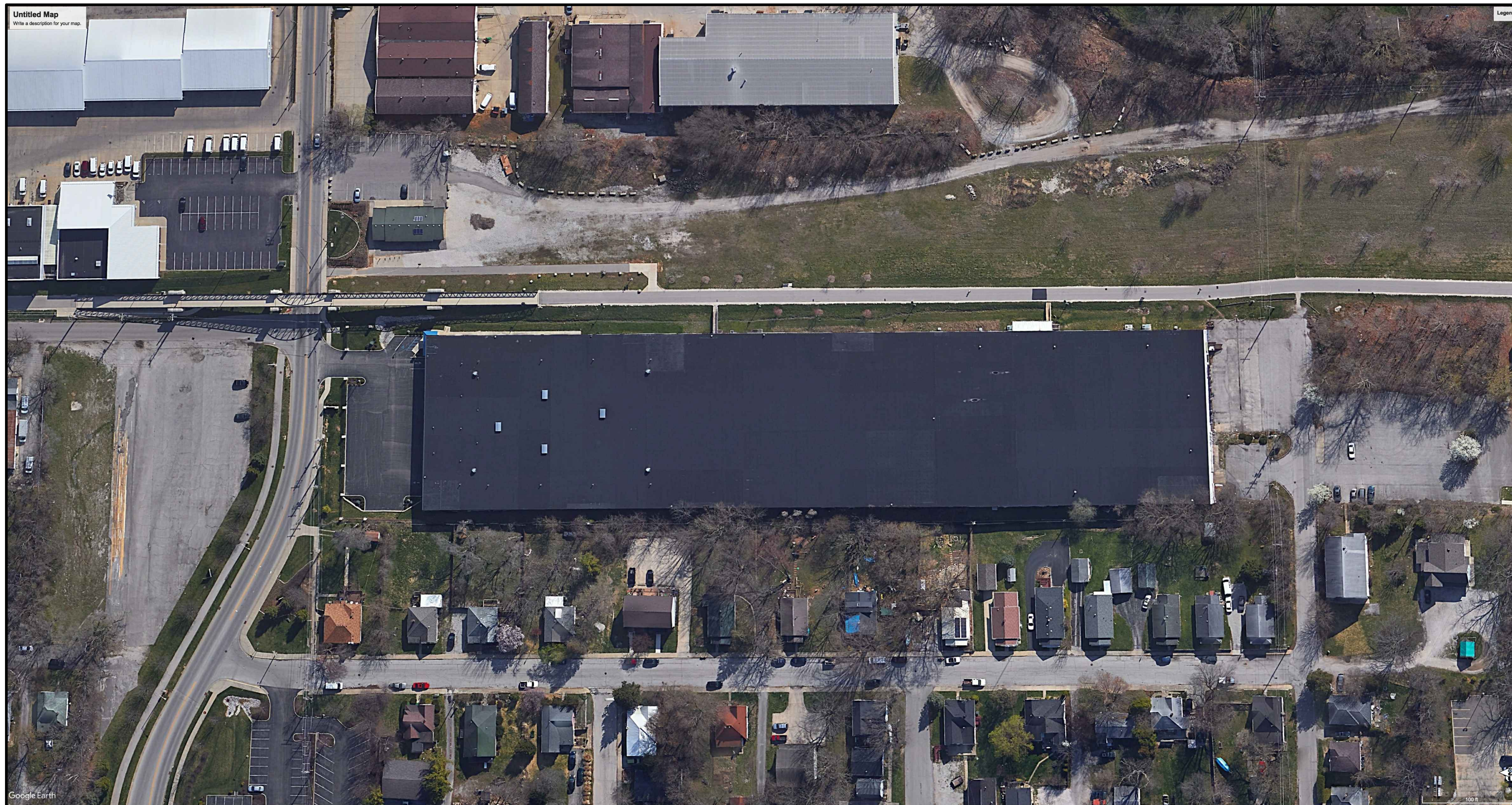
A EXIST. CONDITIONS PHOTO NTS
