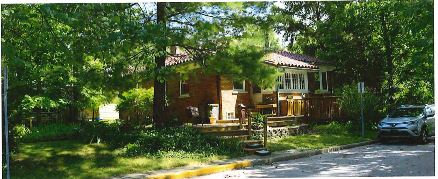
VIEW FROM NORTH-EAST APPROACH ALONG S FACULTY ST.
