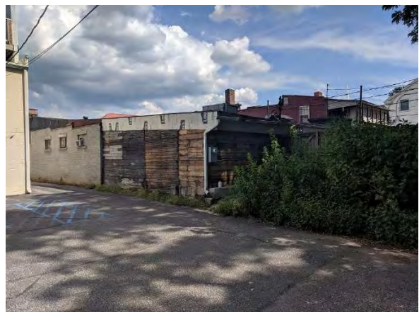
Northwest Façade (exposed wall & roof)
