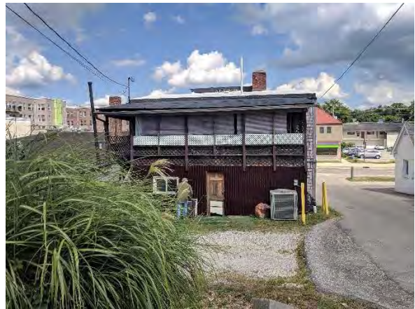
West Façade (porch over storage addition)
