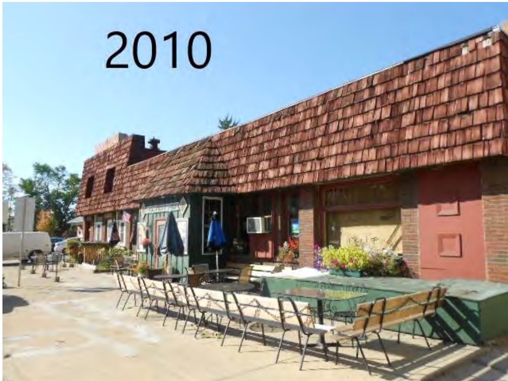
Photo taken in 2010 shows that the lower half of the façade has been restored and windows opened.
