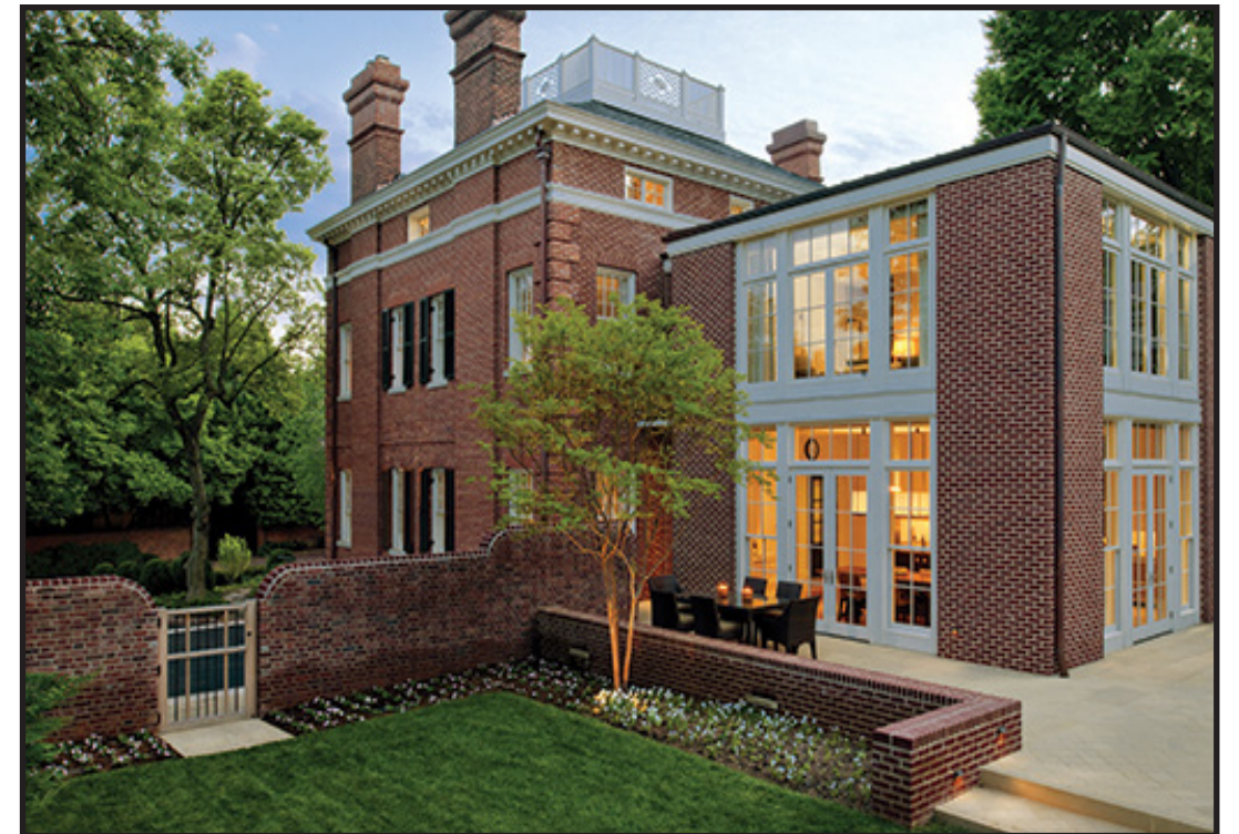
This glass and brick structure is a harmonious addition set back and connected to the rear of the Colonial Revival-style brick house. The addition is Compatible in materials, color, and proportion. It is Differentiated in that it is subordinate to the historic building and does not unify the two volumes into a single architectural whole. Photograph courtesy of the Secretary of the Interior's Preservation Brief # 14.
