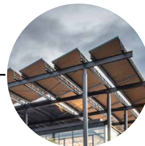
PHOTOVOLTAIC PANEL CANOPY
