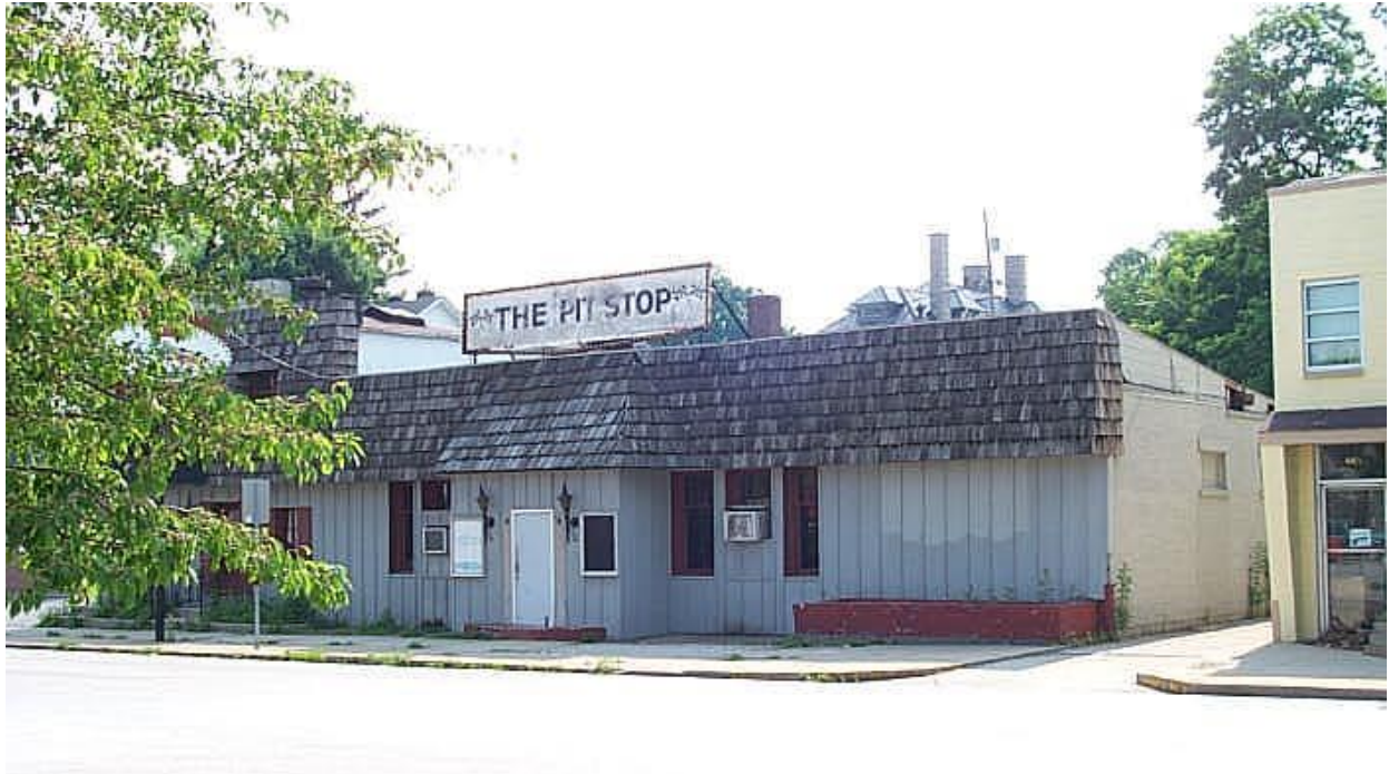
Photo taken in 2001 shows the heavily altered façade.
