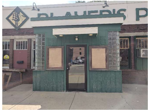
Entry Vestibule (not accessible or original)
