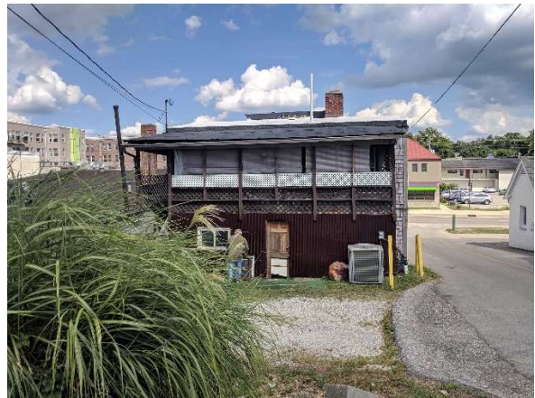
West Façade (porch over storage addition)
