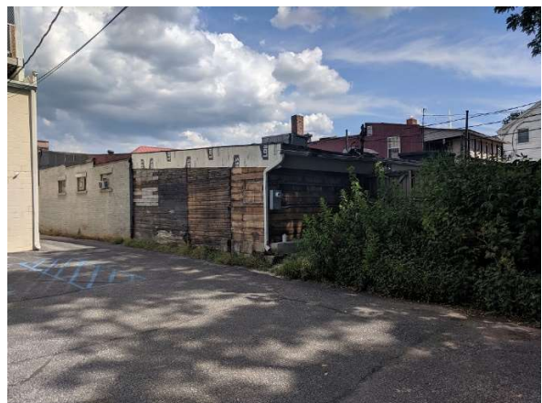
Northwest Façade (exposed wall & roof)
