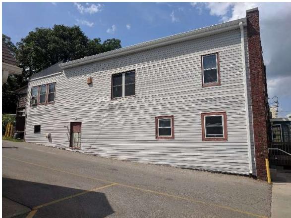
South Façade (hidden exterior condition)
