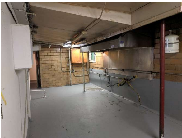
North Building former kitchen
