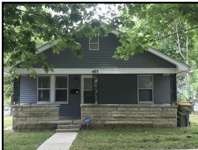
Not recommended: Using ornamental metal porch columns.
