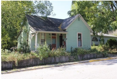
Gabled Ell: 1125 W. 7th Street, c. 1900
