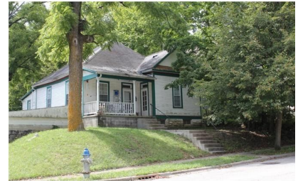
Pyramidal Roof Cottage: 1101 W. 8th Street, c. 1905
