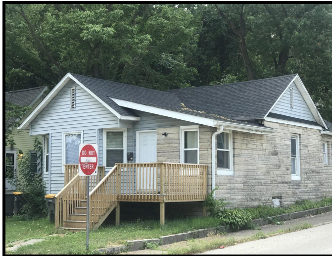
Not Recommended: Porch is enclosed and limestone is used for siding on a wood frame structure originally clad with wood clapboards.
