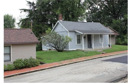
Hall and Parlor: 418 N. Maple Street, c. 1915
