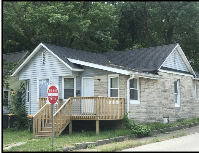
Not Recommended: Porch is enclosed and limestone is used for siding on a wood frame structure originally clad with wood clapboards.
