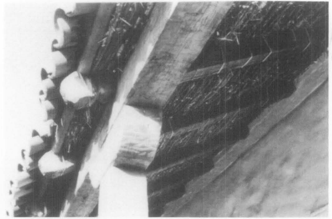
Fig. 10. The underside of this roof on the restored barracks at Santa Cruz Mission reveals the twig sheathing or latia to which the clay tiles were traditionally attached with mud mortar. Photo: Gil Sánchez, FAIA.
