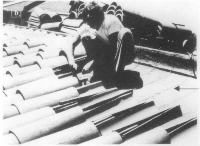
Figure 13 (a-b). These custom-made tapered mission tiles are being attached to the roof using a special system. This consists of twisted 10-gauge brass or copper wires that run up the roof slope through a new treated roof ridge, and down the other side of the roof. These twisted wires are placed about 12" (30.5cm) apart, and diamond shapes are twisted into them every 6" (15cm). The vertical wires are secured with 10-gauge copper or brass anchors approximately every 4' (1.22m) on center depending on the roof slope. Although these tiles would have originally been laid in mud mortar, this method of attachment is particularly successful in seismic areas. The random placement of the tiles accurately replicates the pattern traditionally used on the early missions. Photos: Gil Sánchez, FAIA.
