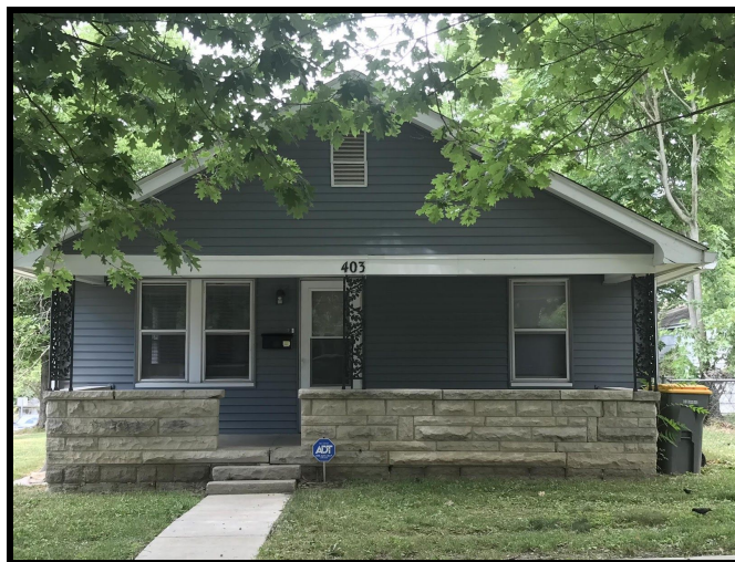
Not recommended: Using ornamental metal porch columns.
