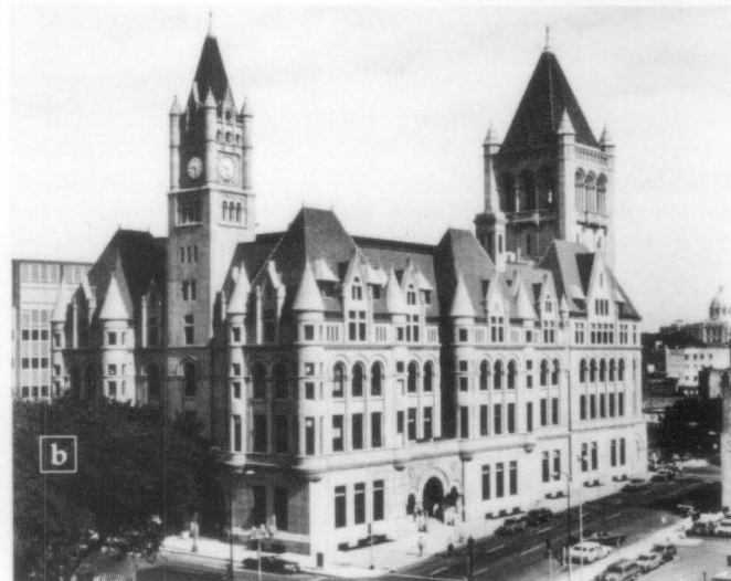
Figure 5. (a) Clay tile was a popular roofing material during the Romanesque Revival period, not only for residential structures including these rowhouses in the Dupont Circle Historic District in Washington, D.C., and designed and built by Thomas F. Schneider between 1889-1892, but also for large-scale public buildings such as (b) the Old Federal Courts Building (1894-1901) in St. Paul, Minnesota, designed by Willoughby J. Edbrooke. Photo: (a) Anne Grimmer, and (b) Winsor/Farcy Architects.
