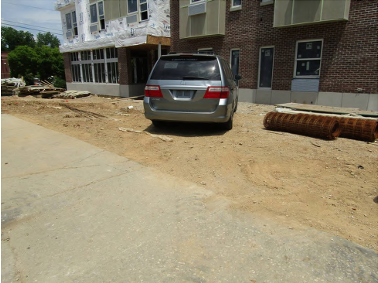
Figure 1: Tracking of sediment onto sidewalk along N. College Ave.
