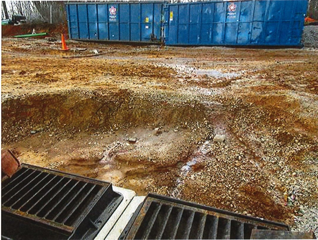
Figure 15: Unknown opaque white liquid seeping from dumpster area directly into the storm drains.
