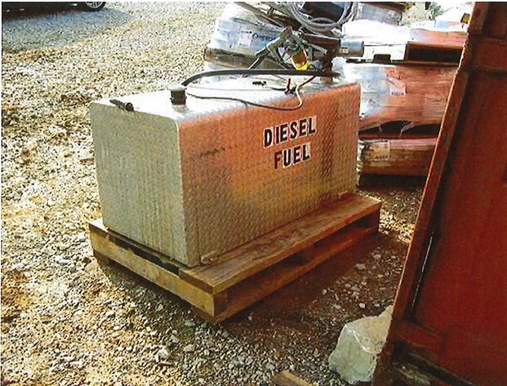
Figure 13: Inappropriately stored fuel tank. This tank should not be sitting, on a slant, on a pallet. There was also no spill kit available.
