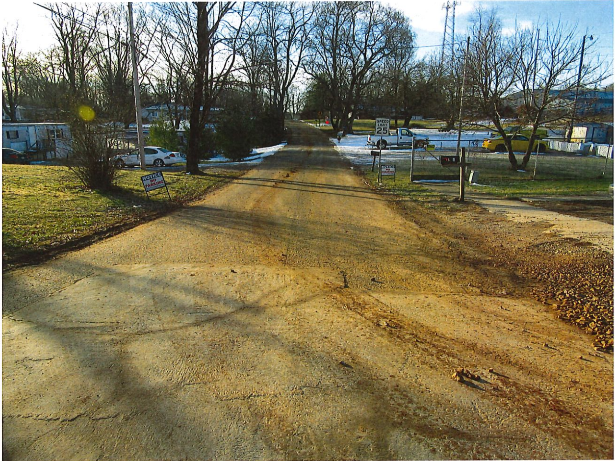
Figure 9: Tracking onto Oolitic.
