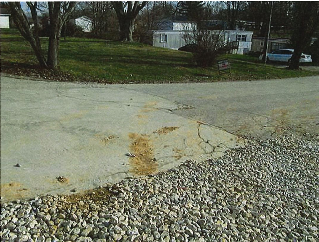
Figure 2: Tracking of sediment onto Oolitic Drive.
