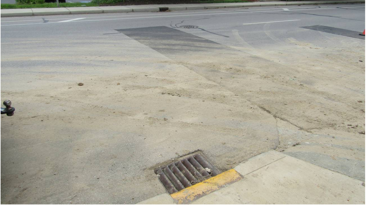
Figure 7: Tracking onto N. Walnut St and inlet without protection.
