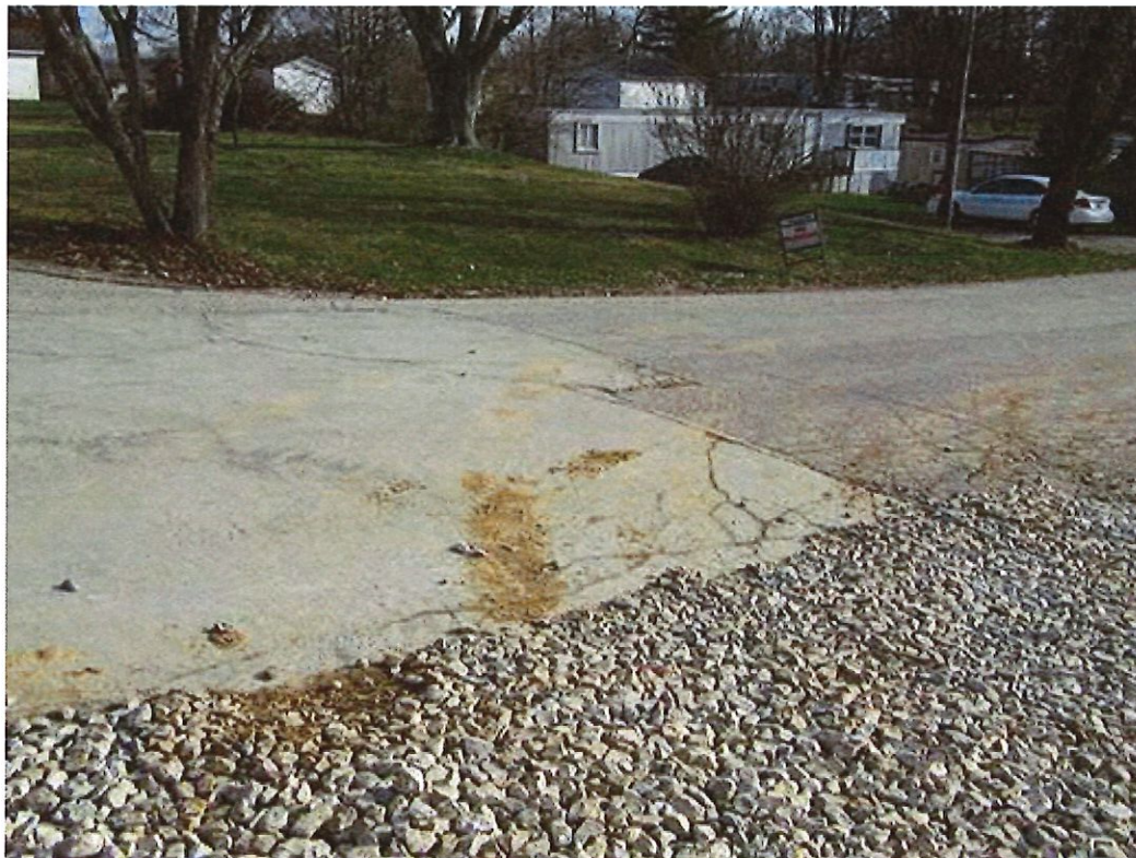
Figure 2: Tracking of sediment onto Oolitic Drive.
