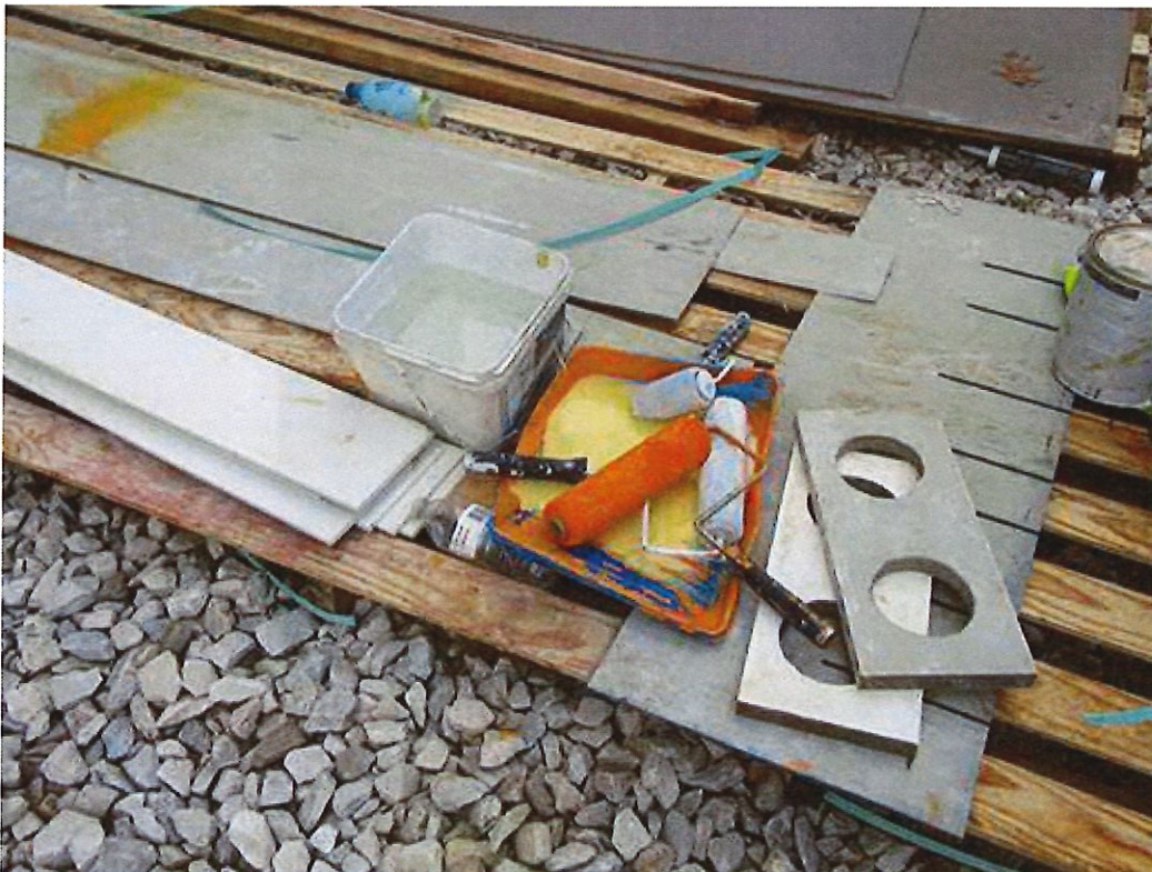
Figure 10: Inappropriately disposed of paint products. These items were left outdoors to collect rainwater.
