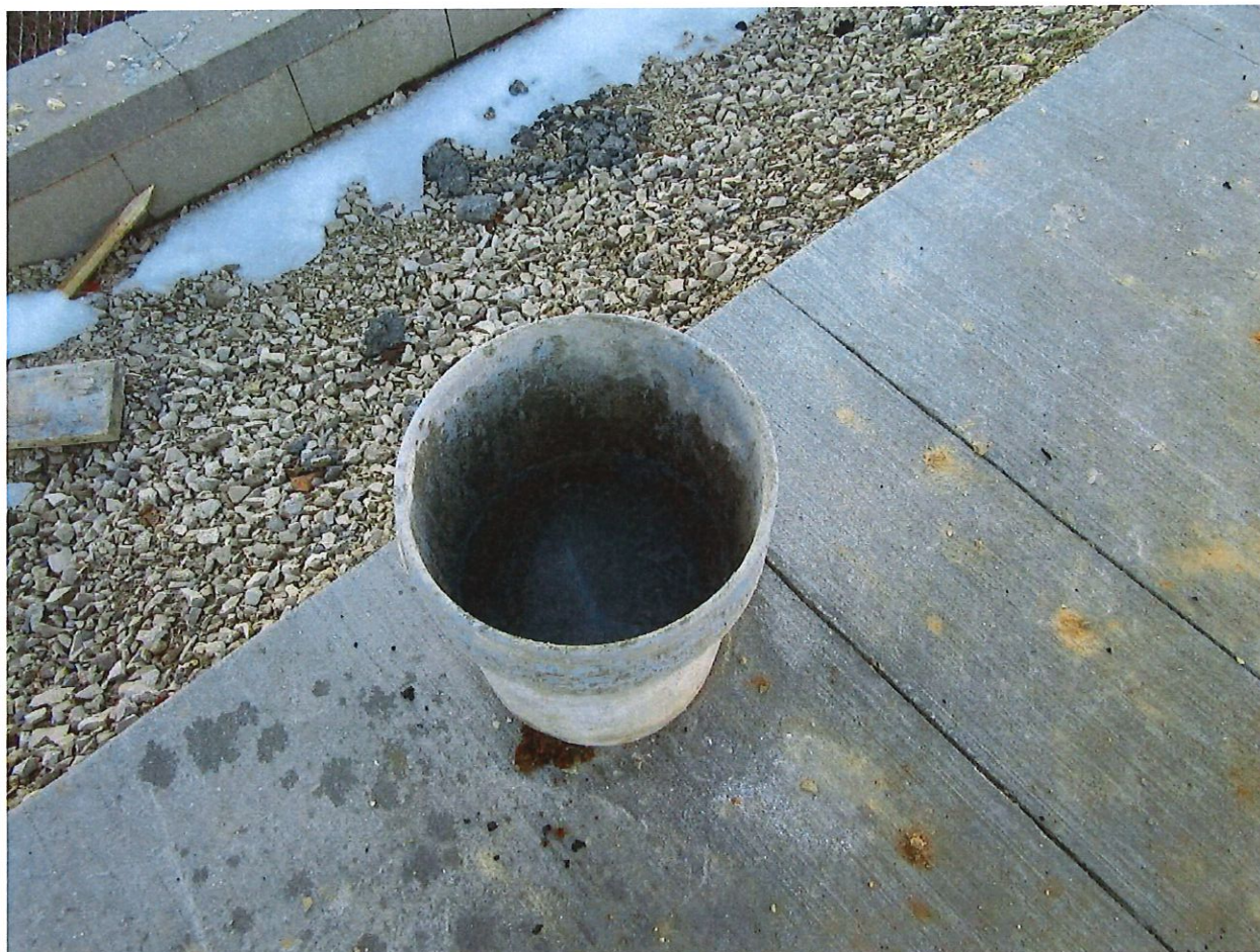
Figure 7: Bucket was used to mix some kind of substance. The substance was not properly disposed of. The bucket was left uncovered to fill with rain water.
