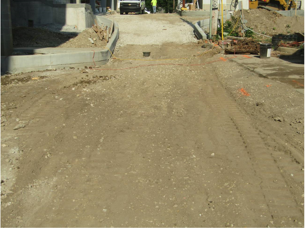
Figure 4: 7/6/2020 - Construction drive/alley that crosses the property.
