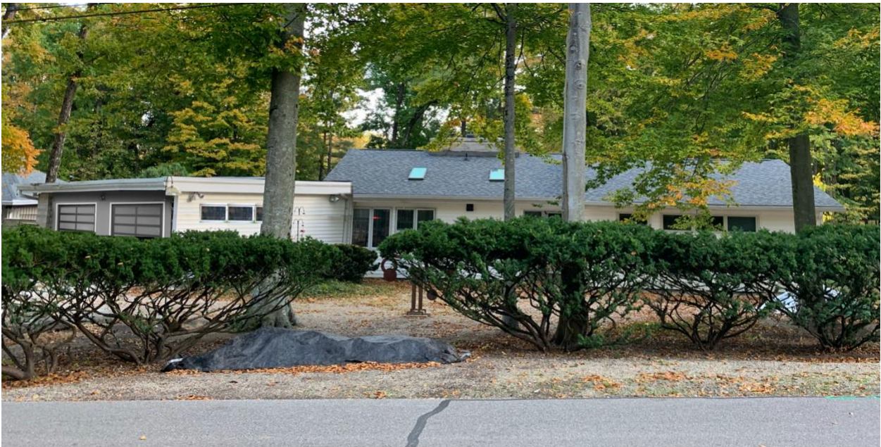
Very rough, amateur photo-shopped rendition of the same view after proposed renovation of carport/garage to illustrate enlarged footprint dimensions and design intention.
