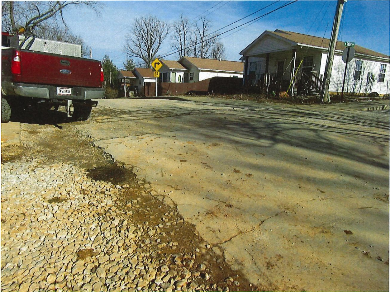
Figure 7: Tracking onto Oolitic.
