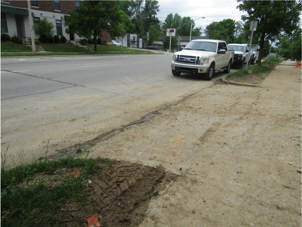
Figure 2: Tracking of sediment onto N. College Ave.
