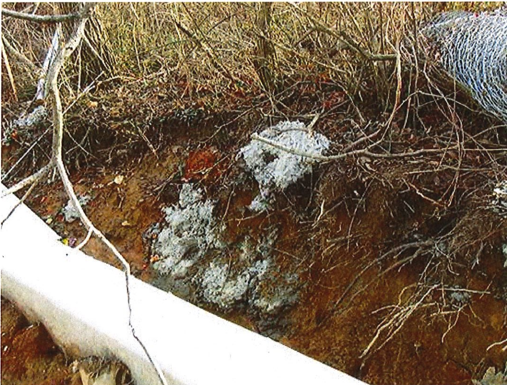
Figure 12: Inappropriately disposed of construction materials.
