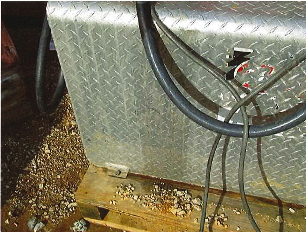
Figure 14: Leaking/spilled fuel running down the sides of the fuel tank and collecting on the pallet.
