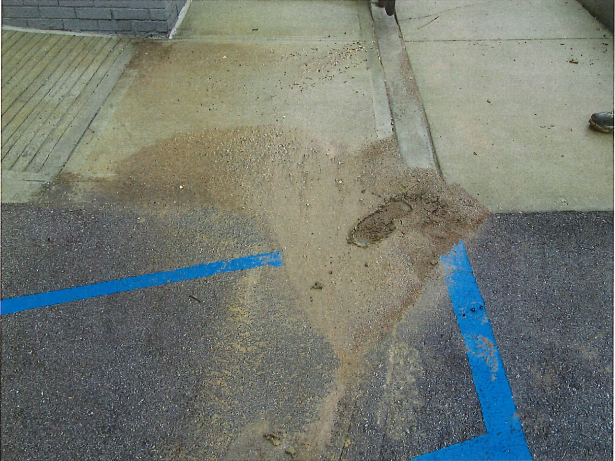
Figure 5: Sediment washed onto neighboring property.
