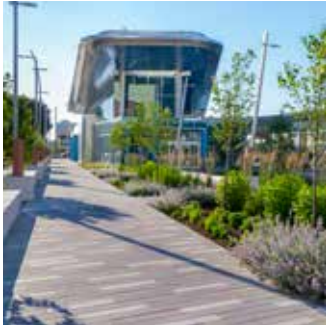
Julia Carson Transit Center, Indianapolis, IN
