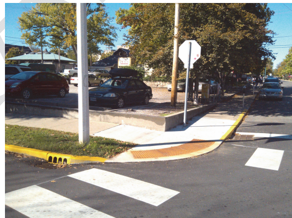
Curb ramps are upgraded in coordination with annual street repaving.
