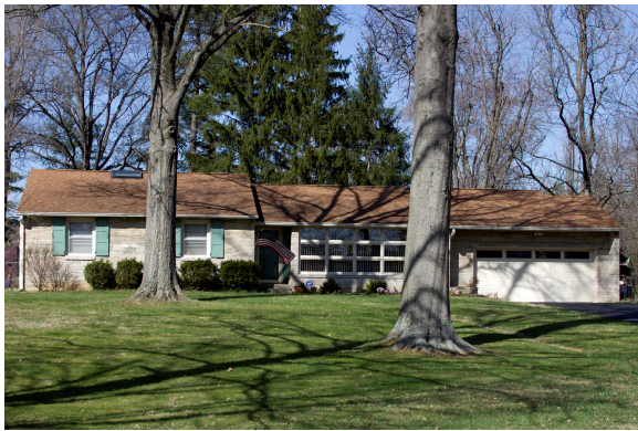
221 Glendora full facade
