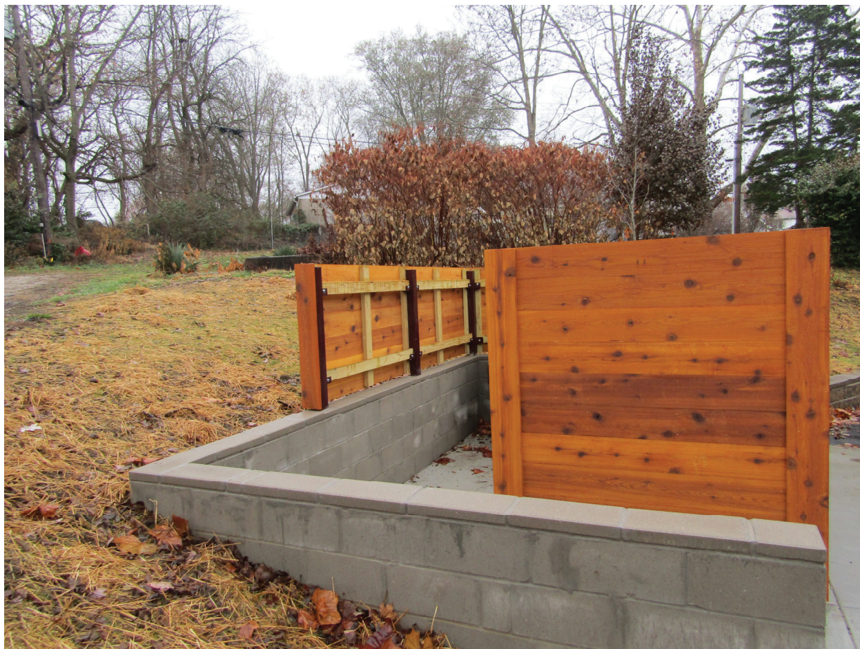
Figure 1: Dumpster is not enclosed on all sides with a minimum 6 foot enclosure.
