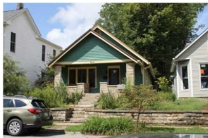
Bungalow: 722 W. 6th Street, c. 1925
