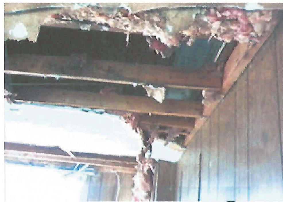
EAST ROOM CEILING (14)
