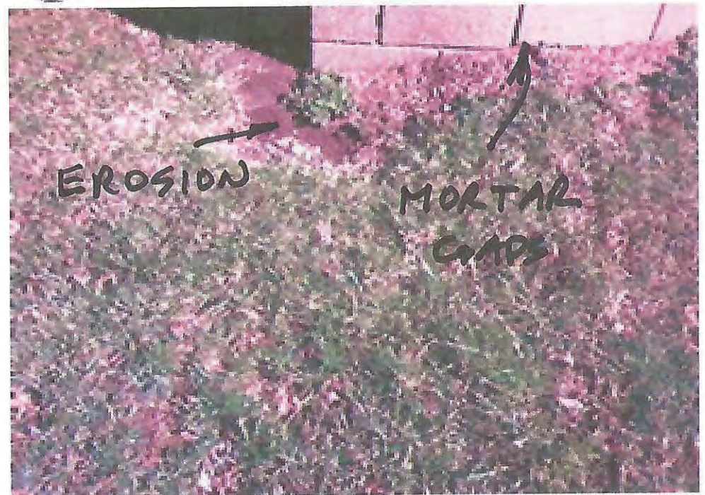
NORTHWEST CORNER ④
