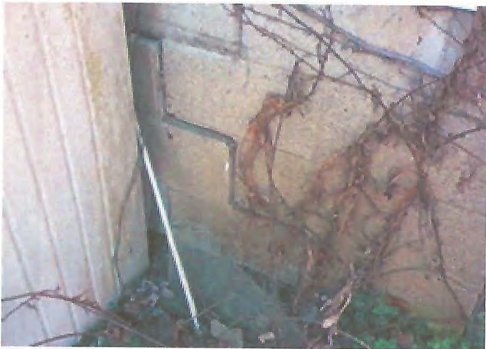
NORTH END - EAST WALL (9)
