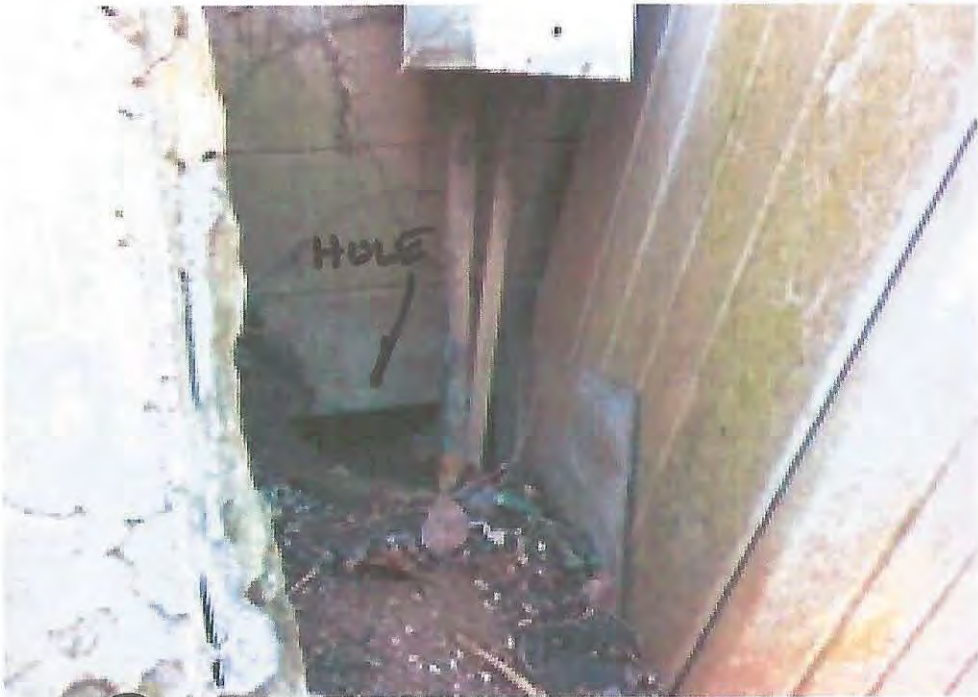
① EAST FOUNDATION WALL
