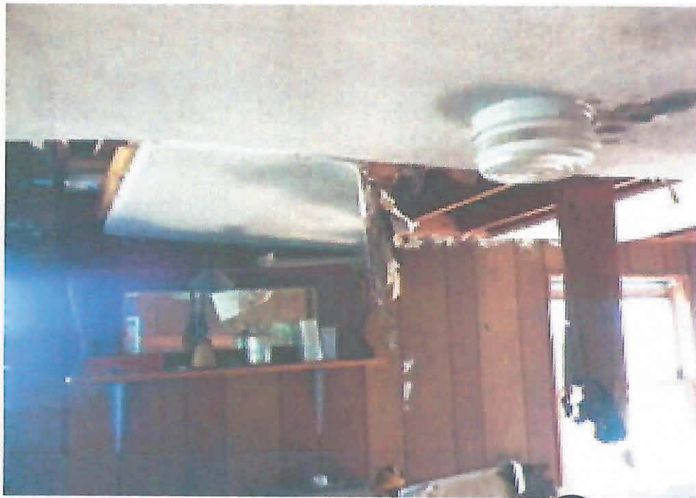
EAST ROOM CEILING (13)
