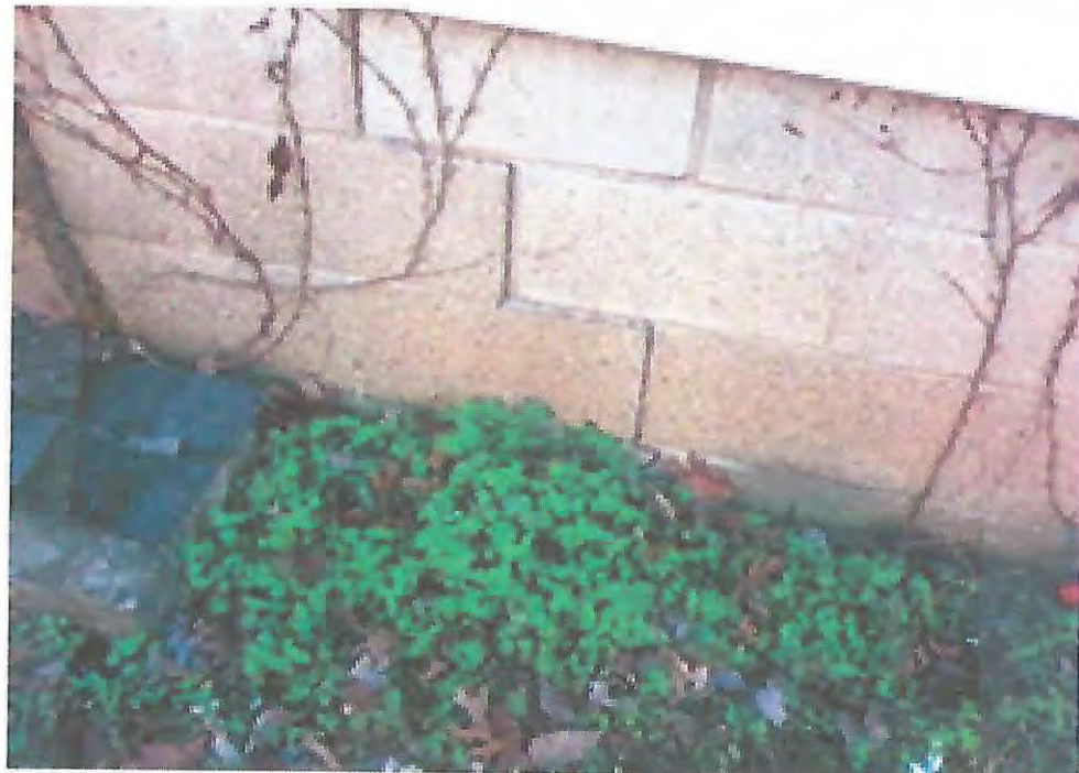
NORTH WALL - EAST END (10)
