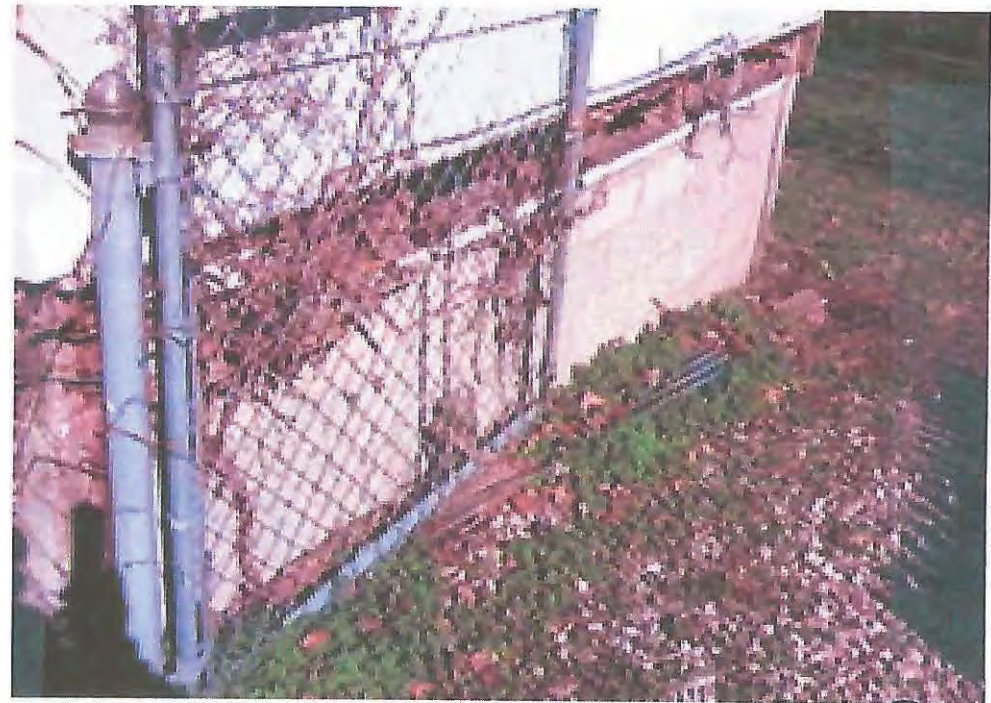
SOUTH WALL - EAST ADDITION 6
