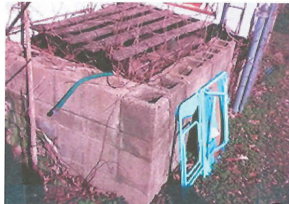
SOUTH PORCH FOUNDATION (16)
