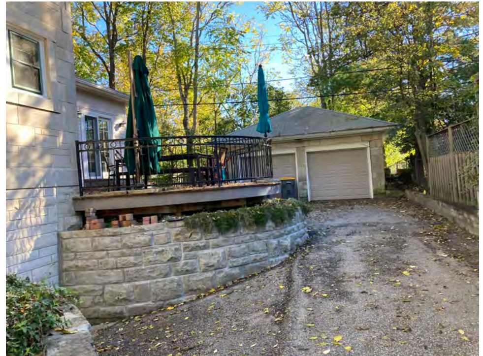
1014 E. Wylie Street - Garage Detail
