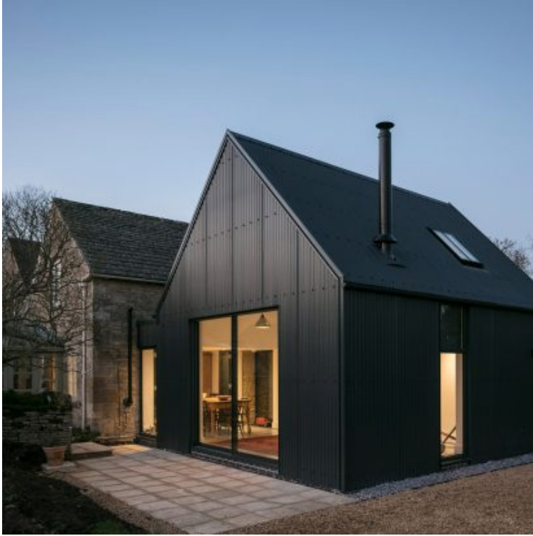
Figure 11 Corrugated metal siding; an important part of Indiana vernacular architecture, but not currently allowed in Bloomington.
