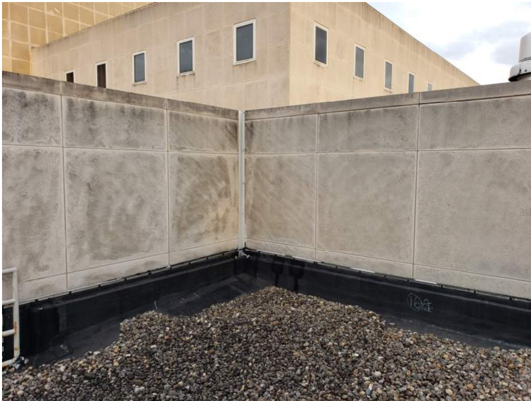
1992 Hospital Addition Constructed on Northwest Corner of Kohr Building Roof
