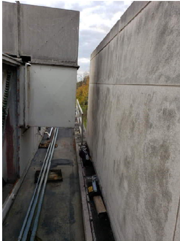
1992 Hospital Addition Constructed on 1981 Stair Tower Roof
