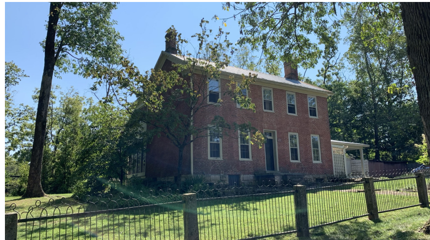
FRONT ENTRY FACADE
