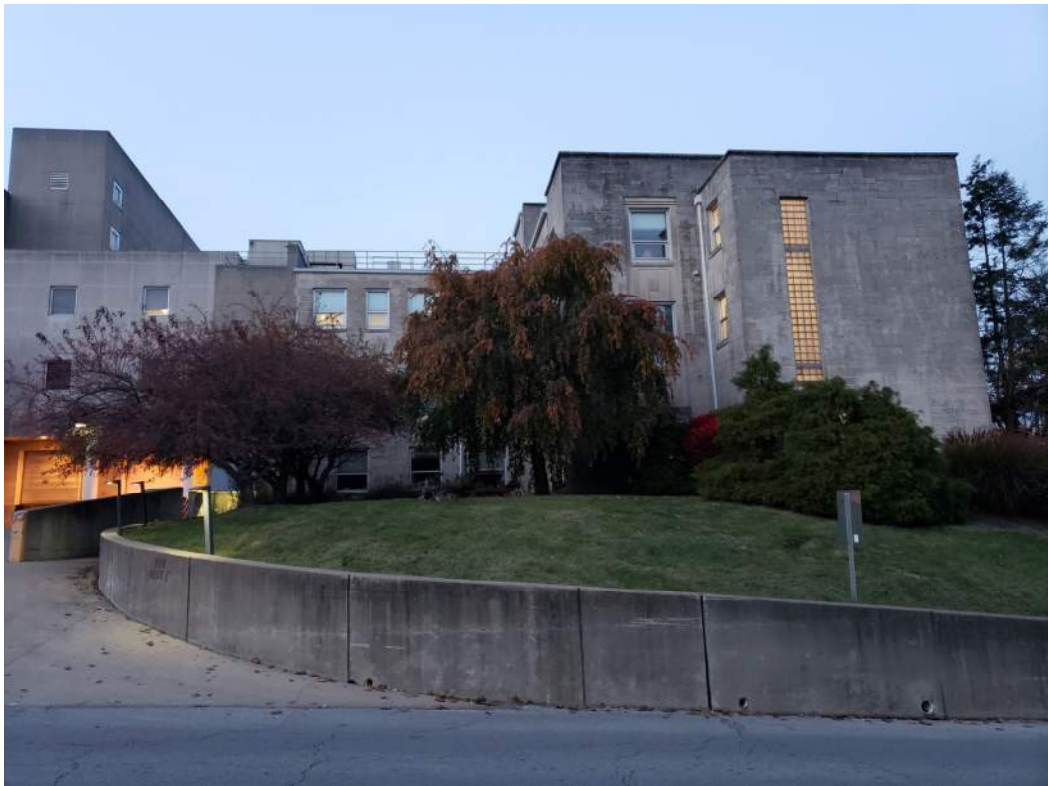
Kohr Building – South Exterior Façade
