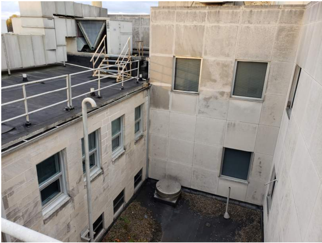
Kohr Building – West Wing – North Facade
