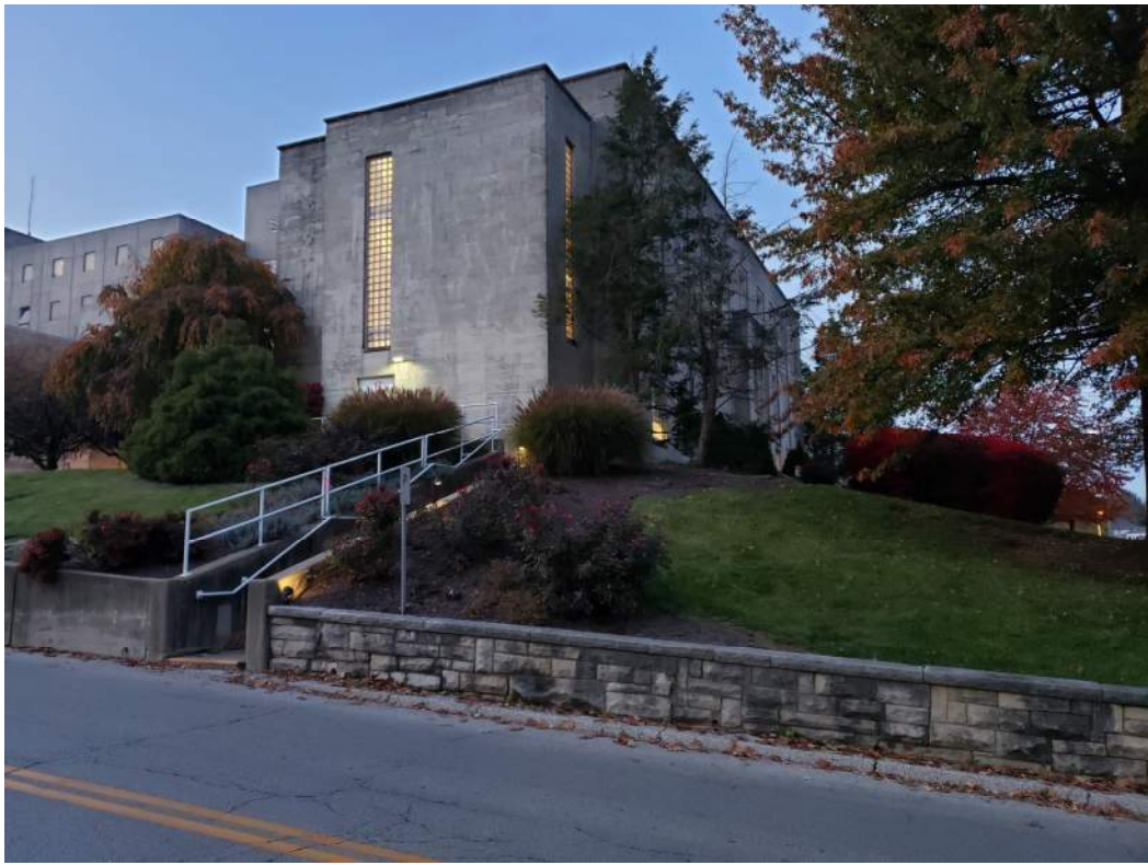
Kohr Building – South-East Exterior Façade
