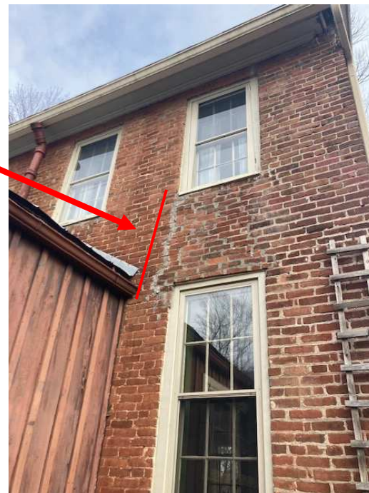
2013 repair to support I-wing (installed 5 helical piers, additional jacks under porch)
