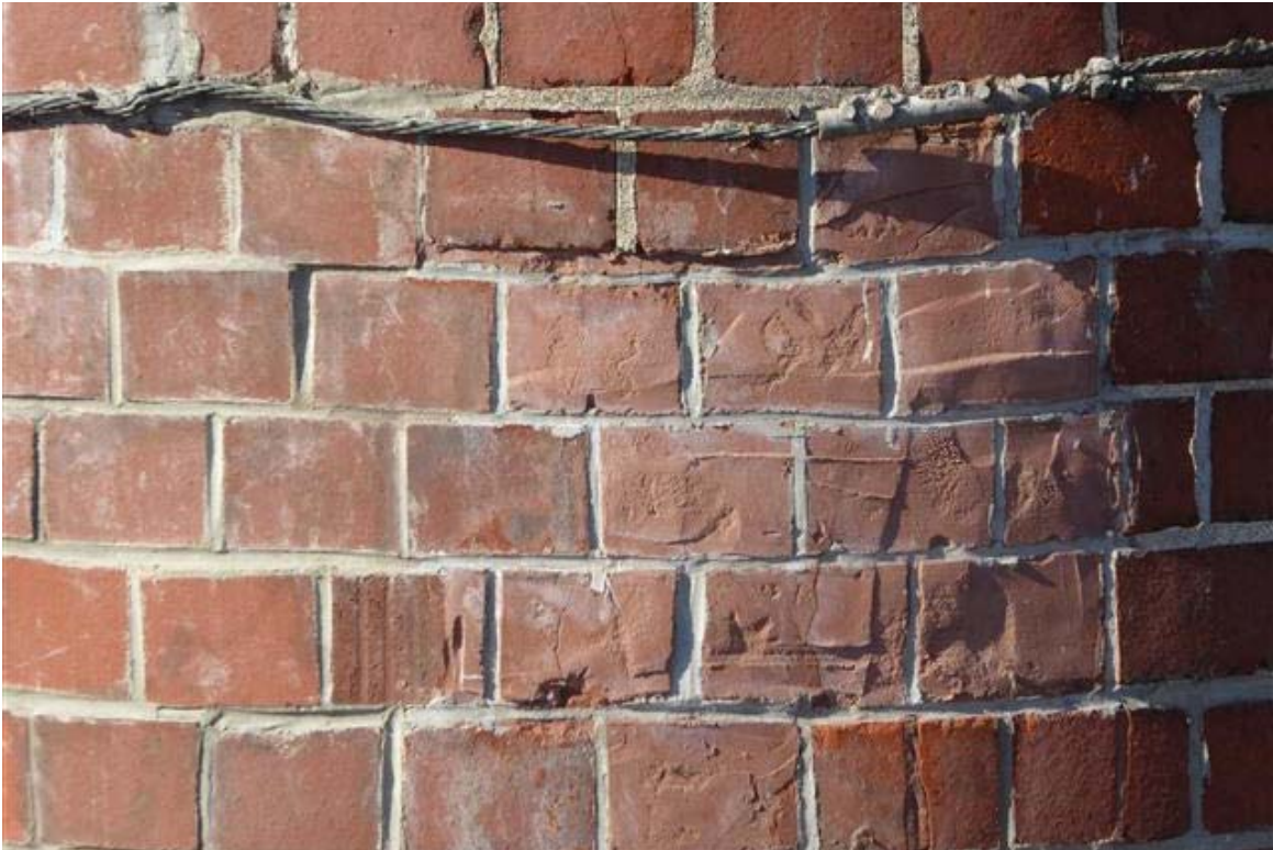
Photo 23 Cementitious patches have been used to replace spalled brick in numerous locations.
