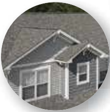
Roofing and Ventilation
