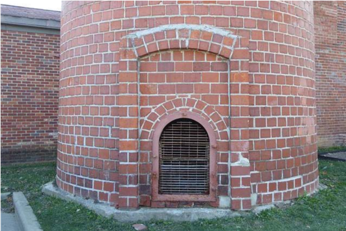
Photo 13 Opening at the base of the stack.
