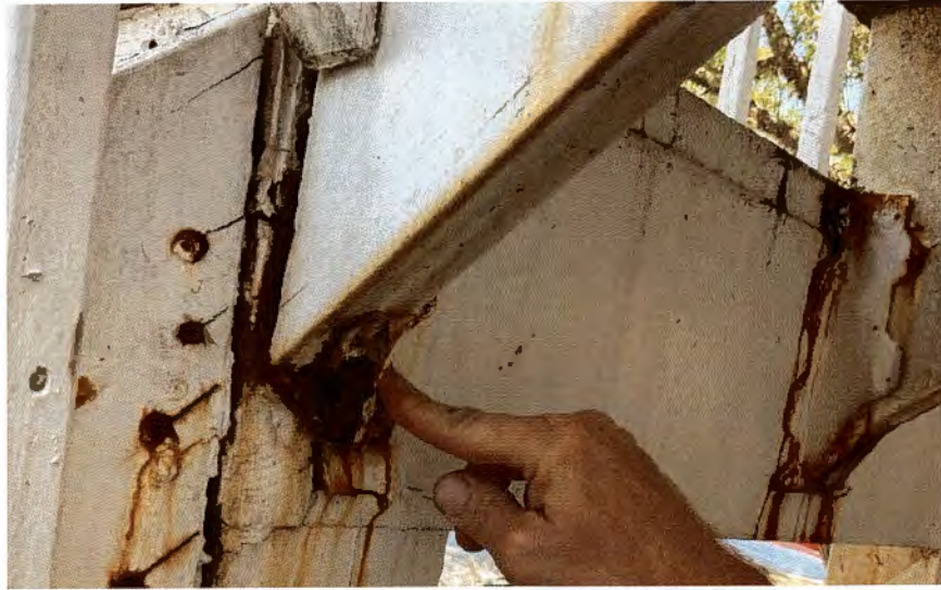
Example of deteriorated joist hanger
