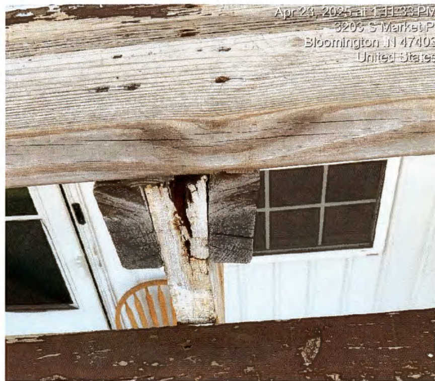
Example of deteriorated stringer
