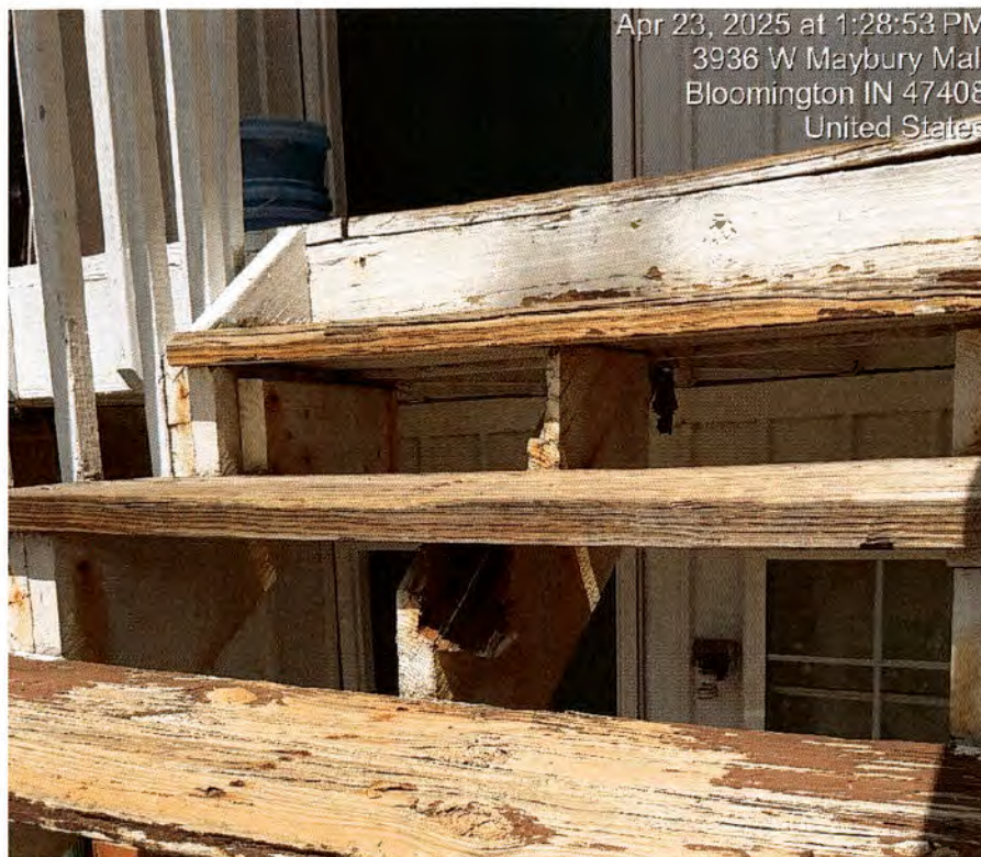
Example of deteriorated stringer
