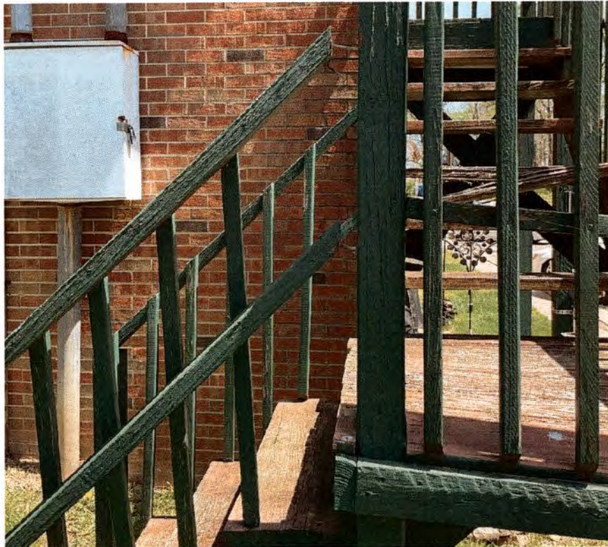
Example of loose handrail and missing spindles
