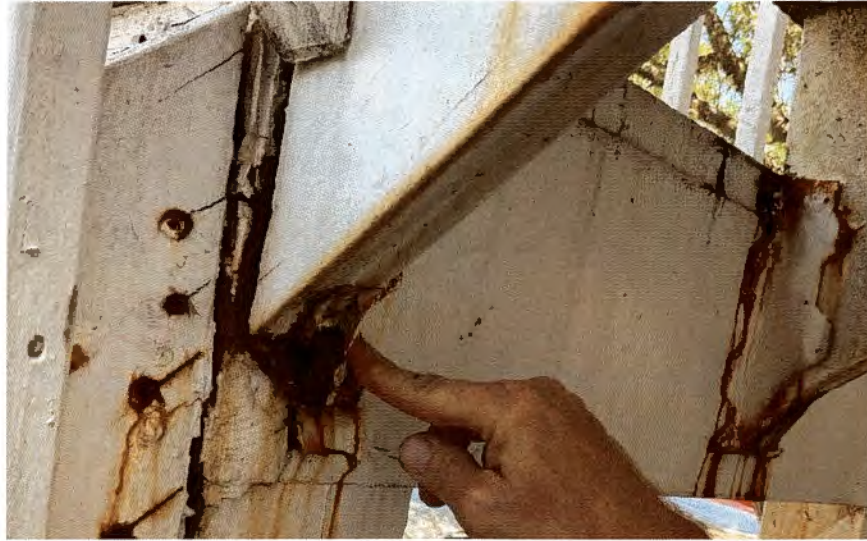
Example of deteriorated joist hanger
