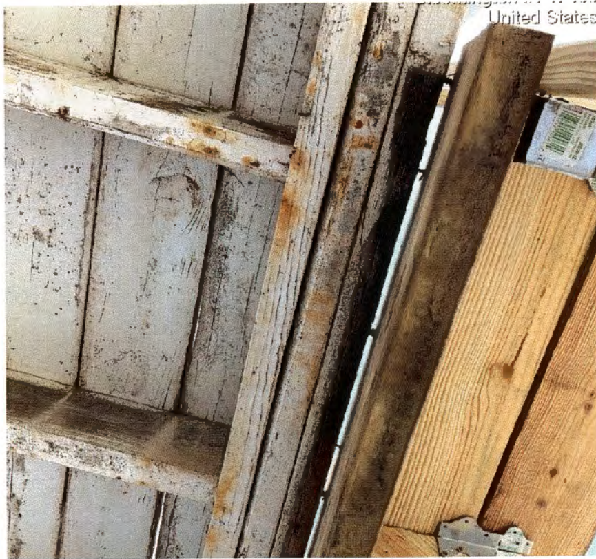
Example of stairs pulling away from upper level walkway
