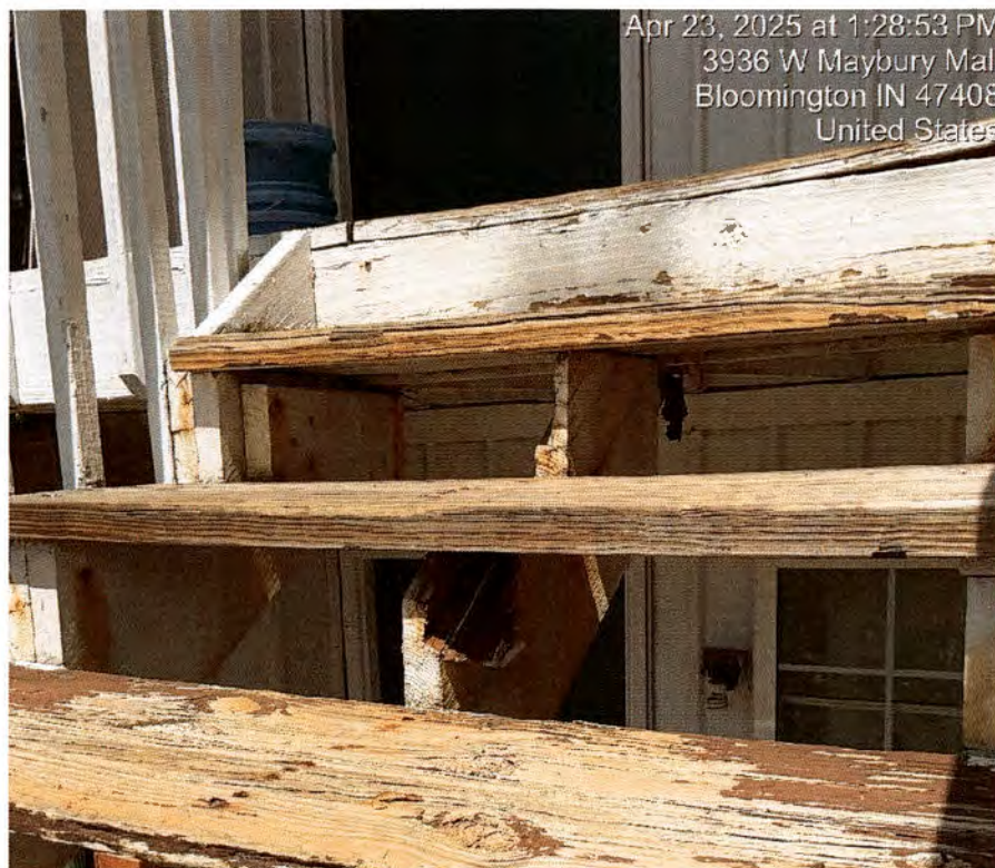
Example of deteriorated stringer
