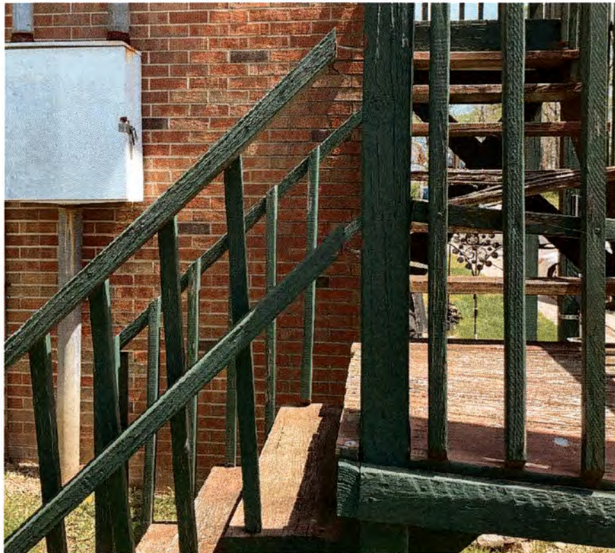
Example of loose handrail and missing spindles
