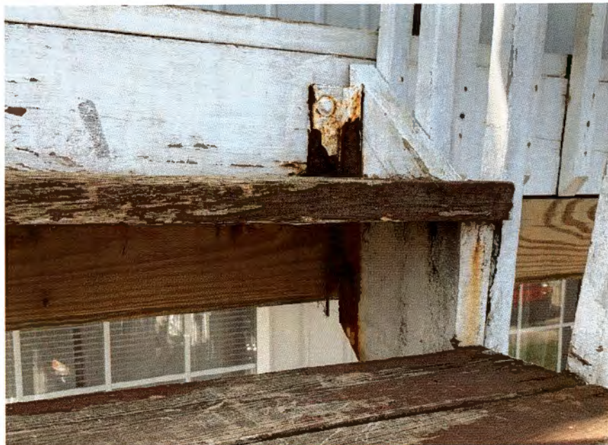
Example of deteriorated brack
