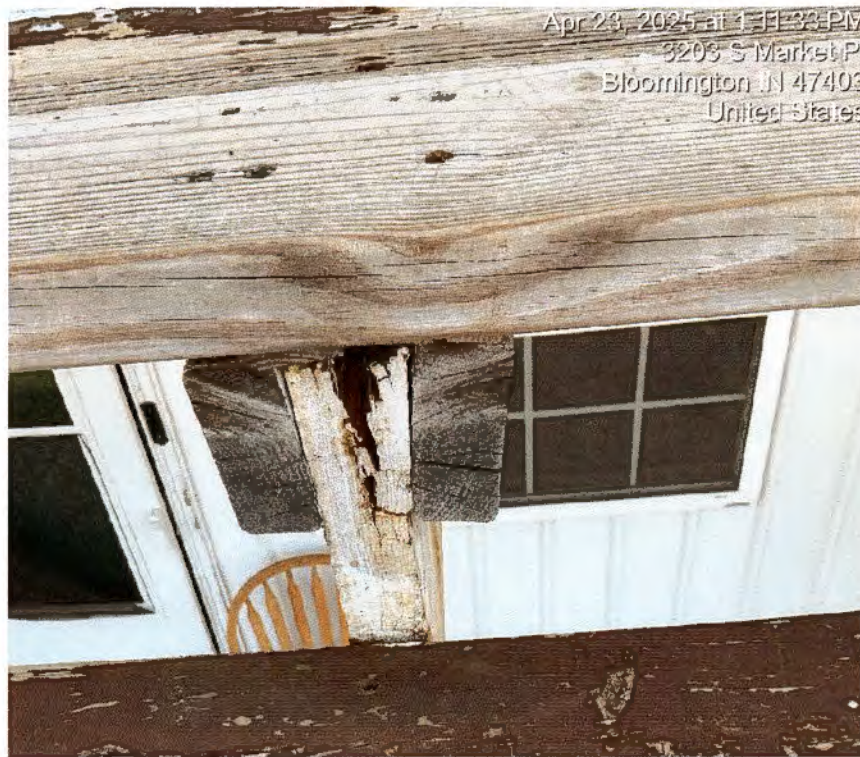
Example of deteriorated stringer
