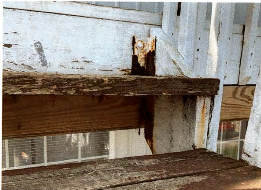
Example of deteriorated brack
