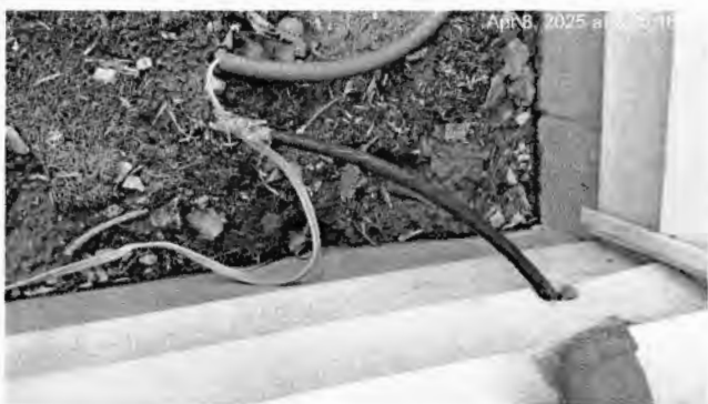
Building 2951 Open Junction Box, exposed wires, disconnected wire, etc.
