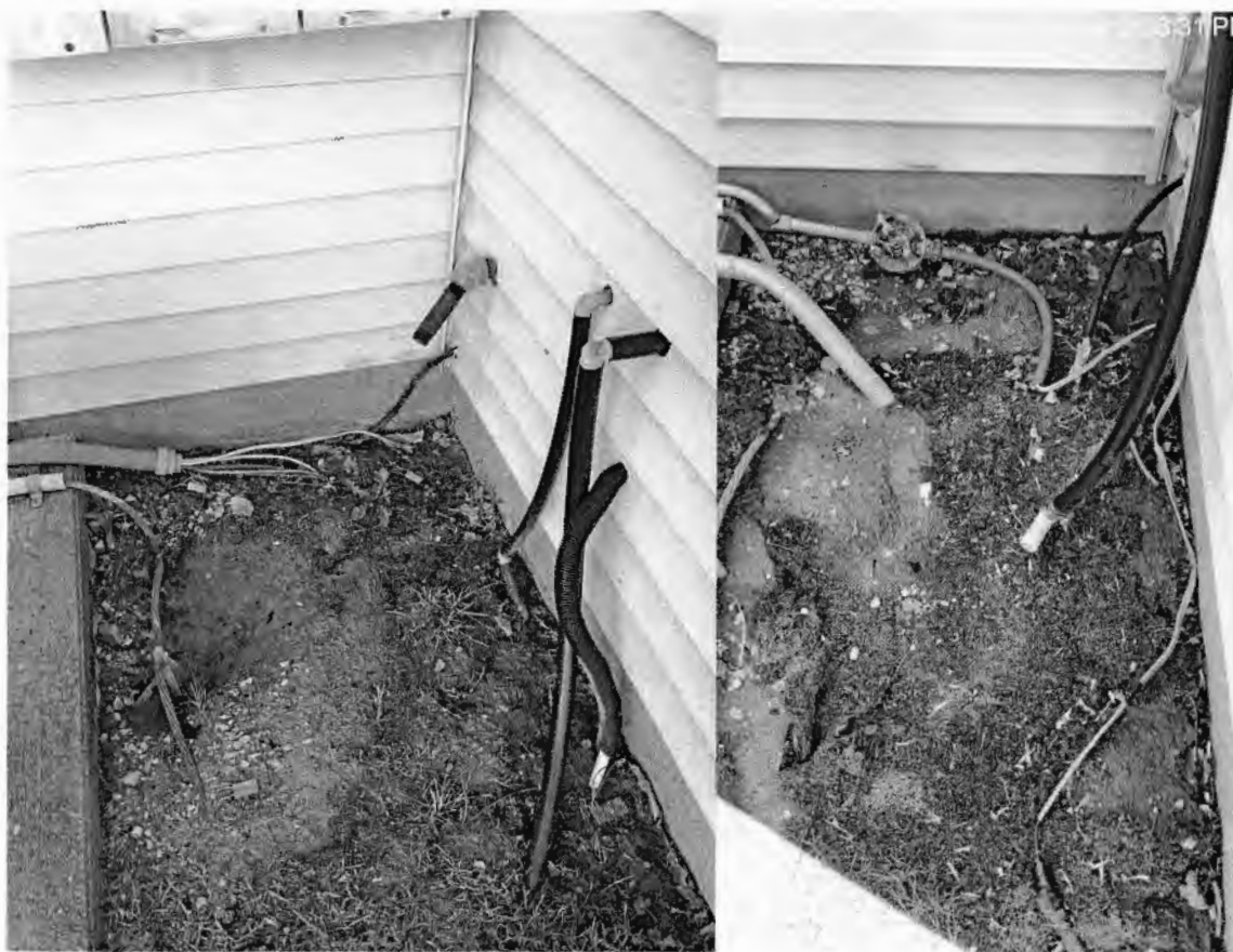
Building 2951 Open Junction Box, exposed wires, disconnected wire, etc.
