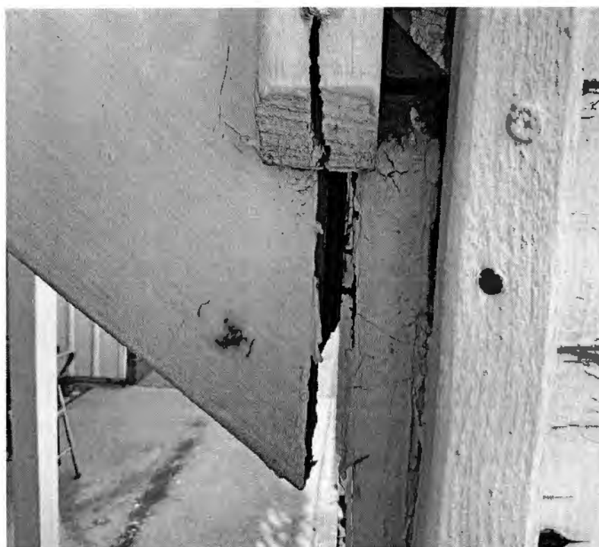
Example of stairs pulling away from upper level walkway
