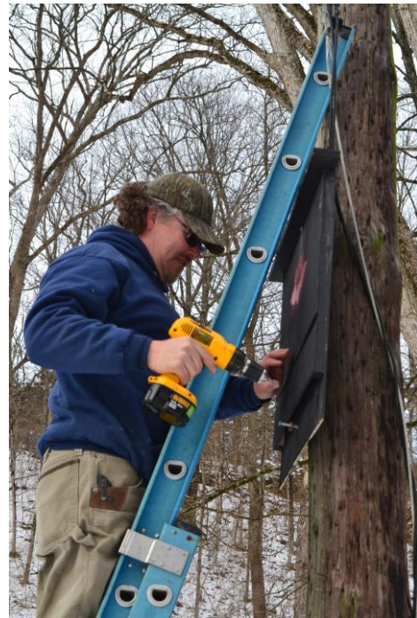
Installing a bat box at the Goat Farm
