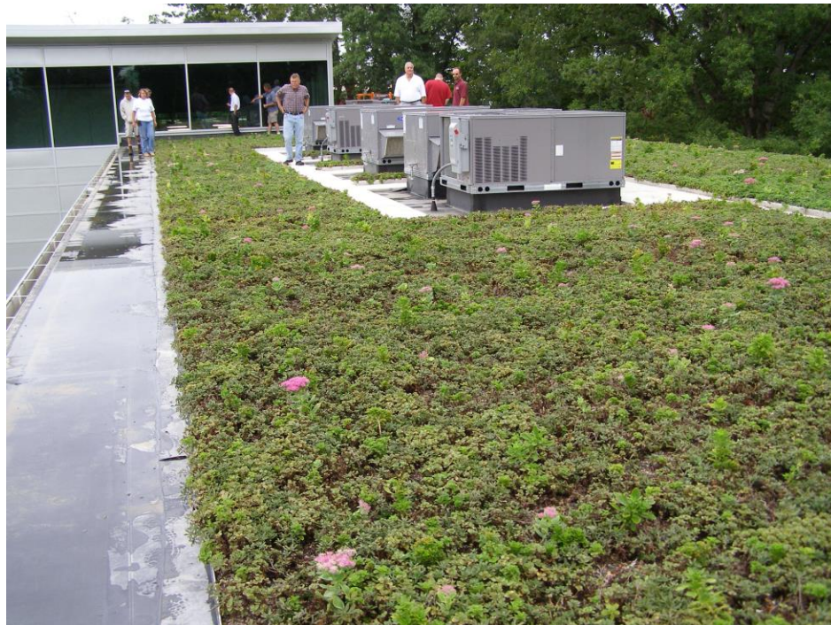
Green roofs are more energy efficient than traditional roofs, reduce stormwater runoff, improve air quality, and promote biodiversity
