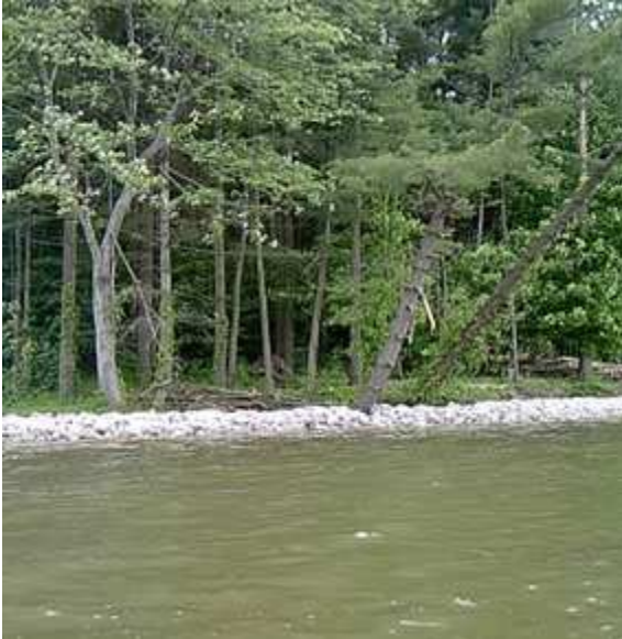
Figure 2 – White stone riprap installed along the shoreline of Lemon Lake. Riprap creates a more natural appearance along the edges of waterbodies than solid retaining walls, provide habitat for aquatic life, and protects the shoreline from erosion. (Photo credit: Lake Lemon Conservancy District).
