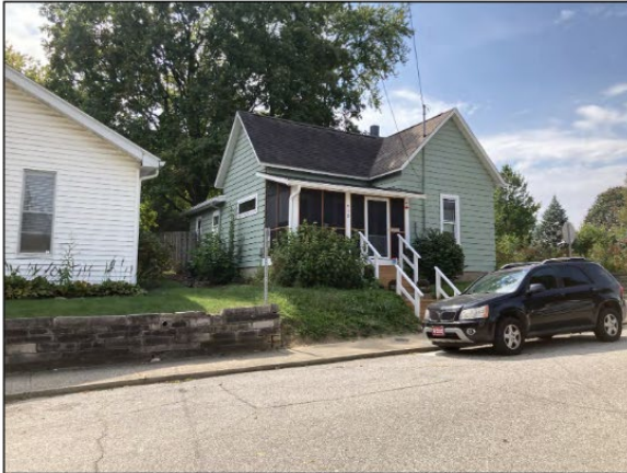
Existing North/Main Facade (no work)
