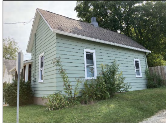
Existing West Facade
