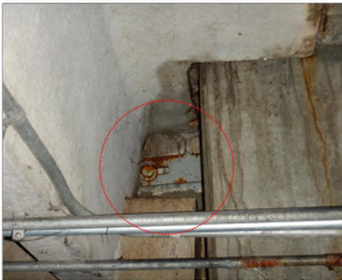
REPAIR ID - 05A
