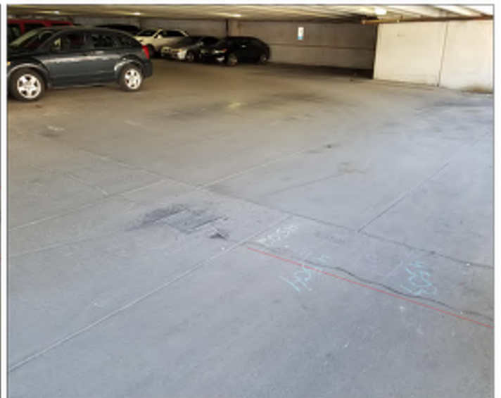
REPAIR ID - 15A
