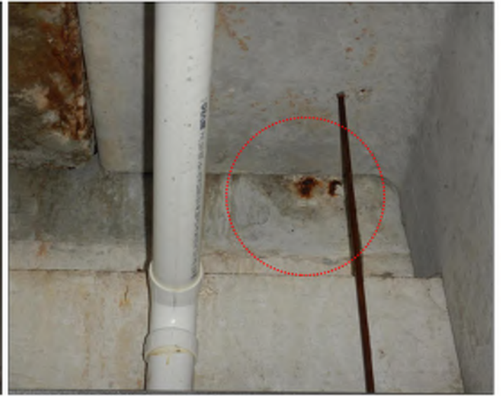
REPAIR ID - 10A
