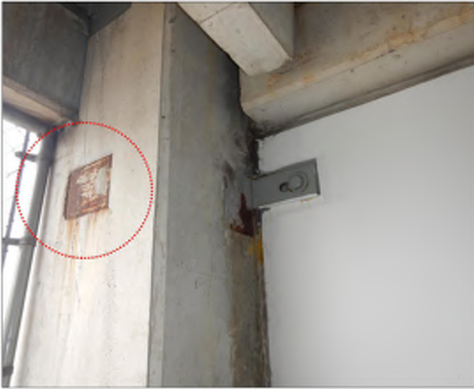
REPAIR ID - 05C
