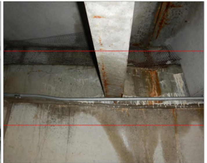
REPAIR ID - 11A
