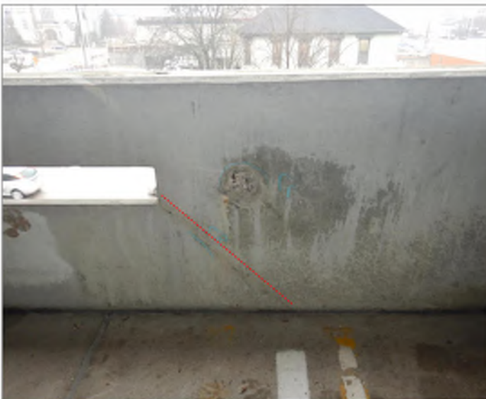
REPAIR ID - 07A
