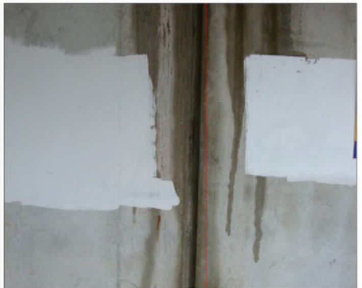
REPAIR ID - 09A
