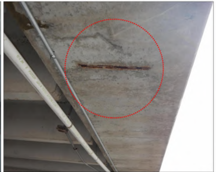
REPAIR ID - 03A
