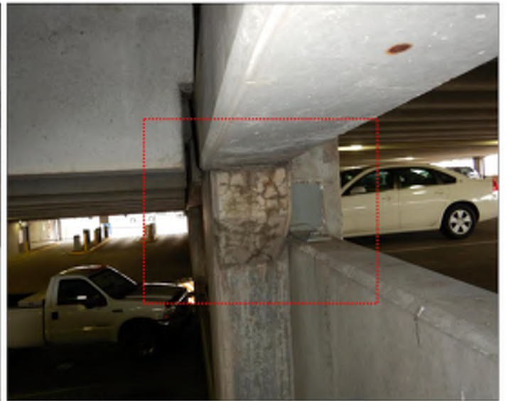
REPAIR ID - 12A
