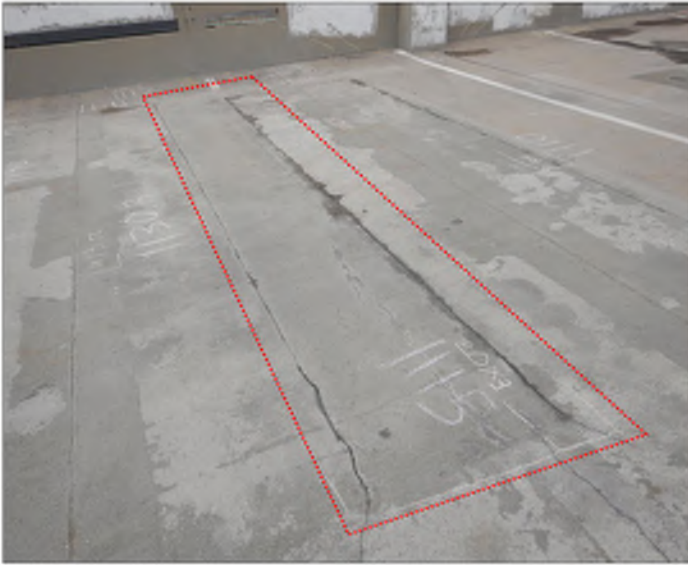
REPAIR ID - 15B
