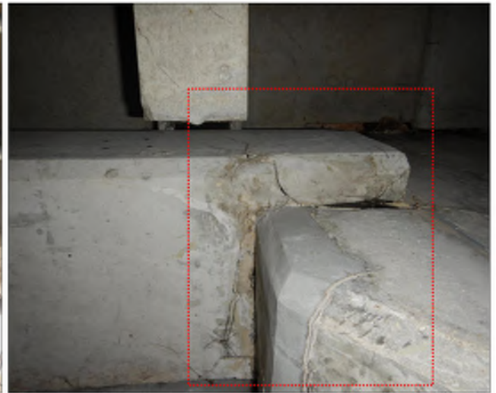
REPAIR ID - 02A
