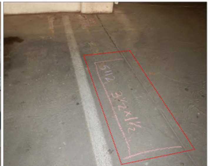
REPAIR ID - 10E-1
