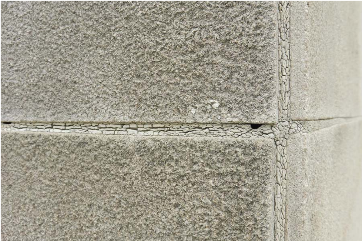
Photo 85 Sealant joints within the limestone panels on the garage...
