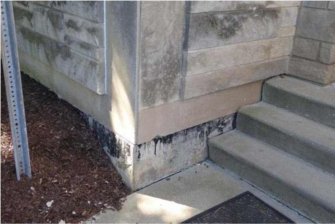
Photo 45 The perimeter basement walls are made of poured concrete.
