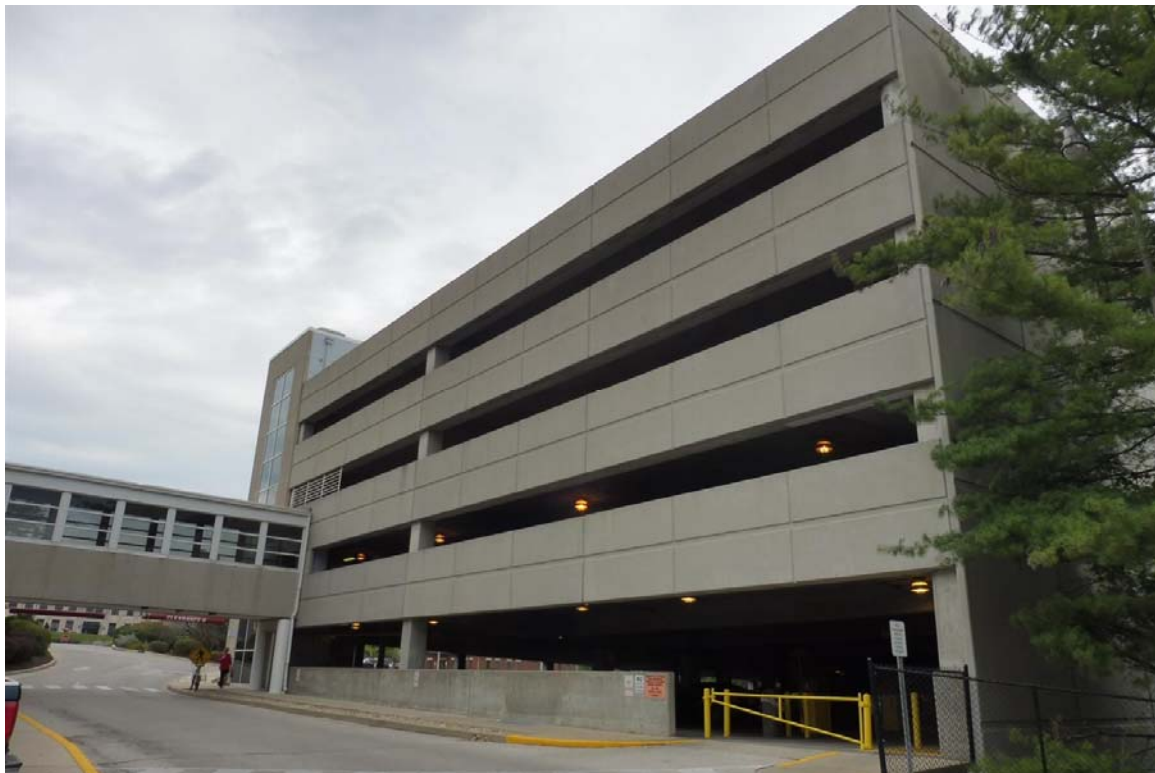
Photo 60 South elevation with connector bridge to hospital.
