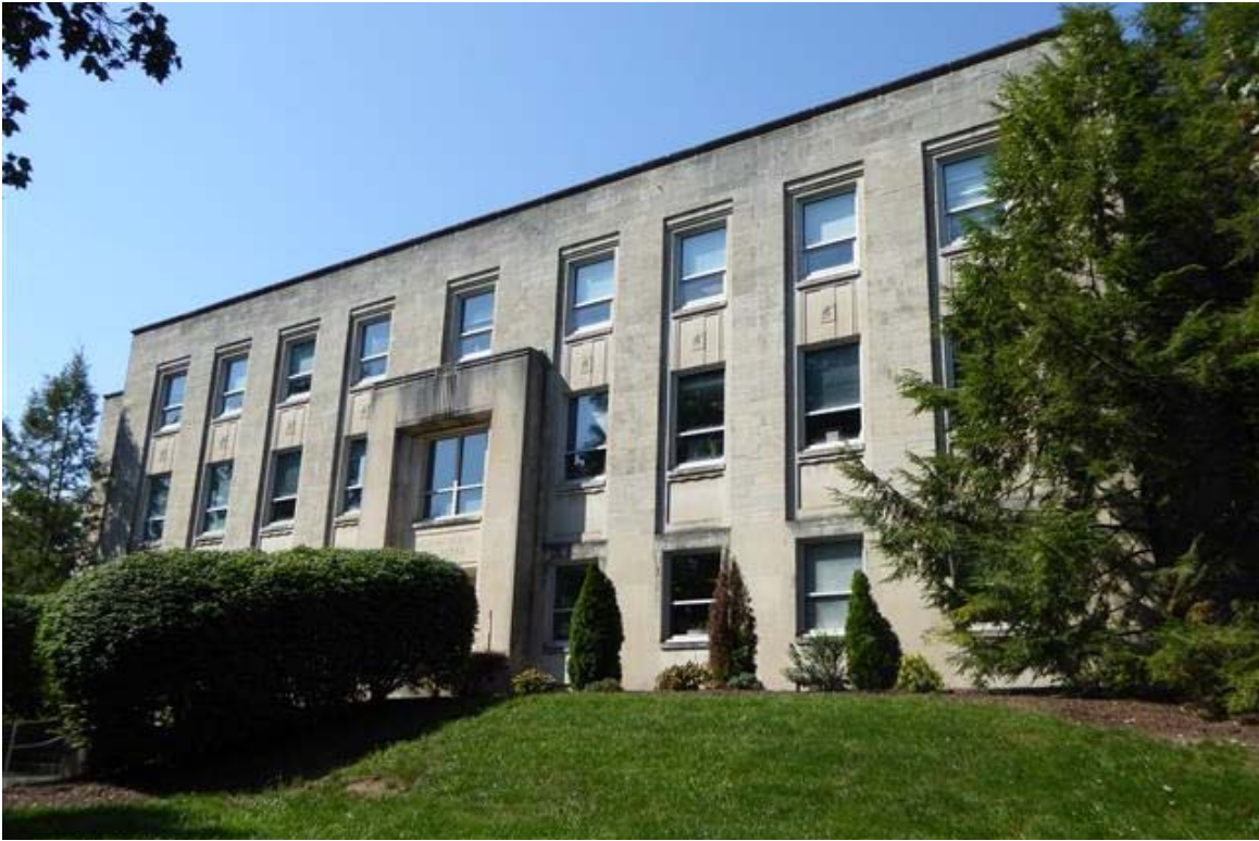
Photo 1 The main elevation faces east.
