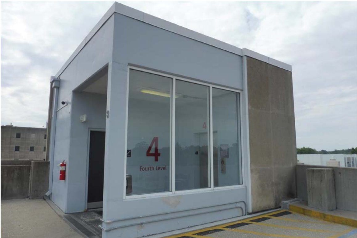
Photo 99 The southwest stair and elevator tower at the roof level.
