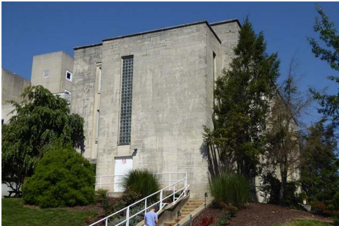
Photo 2 A stairwell extends off the south elevation.
