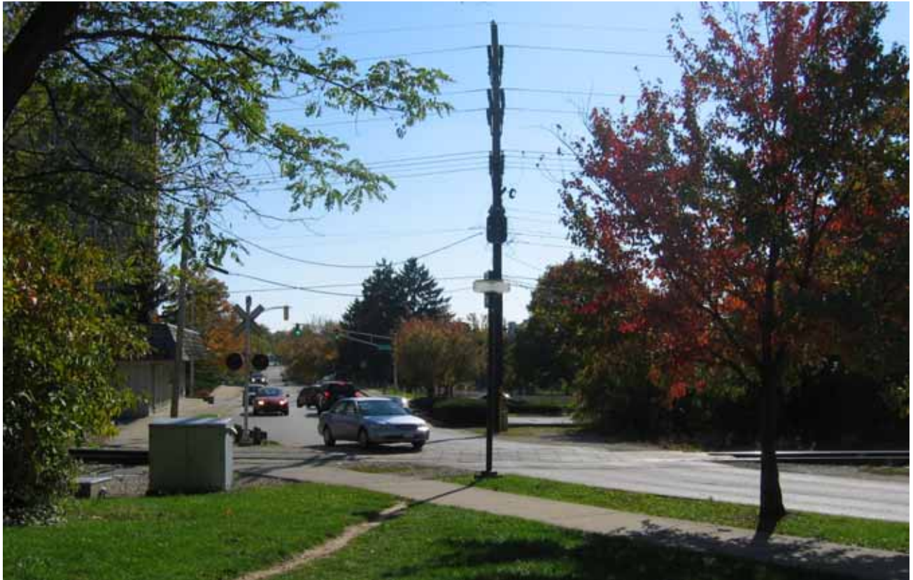
Figure D.17: Union Street at-grade railroad crossing, note the lack of signals.
