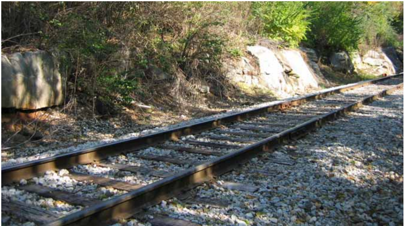
Figure D.12: Railroad track just north of Woodlawn Avenue, note existing cuts into rock.
