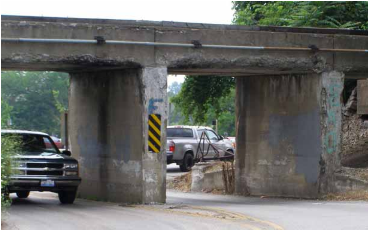
Figure M.1: View of the current condition of the overpass on 10th Street.
