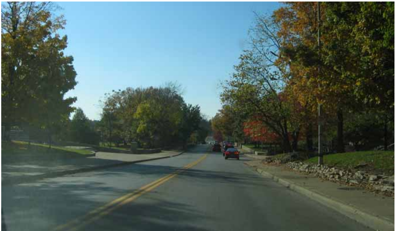
Figure D.6: 10th Street just east of Fee Lane, looking westward.
