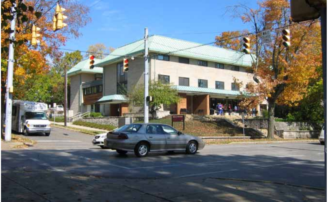
Figure D.9: Intersection of 10th Street and Woodlawn Avenue.
