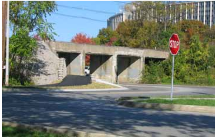
Figure 2: Railroad overpass picture highlighting low clearance and tight turns
