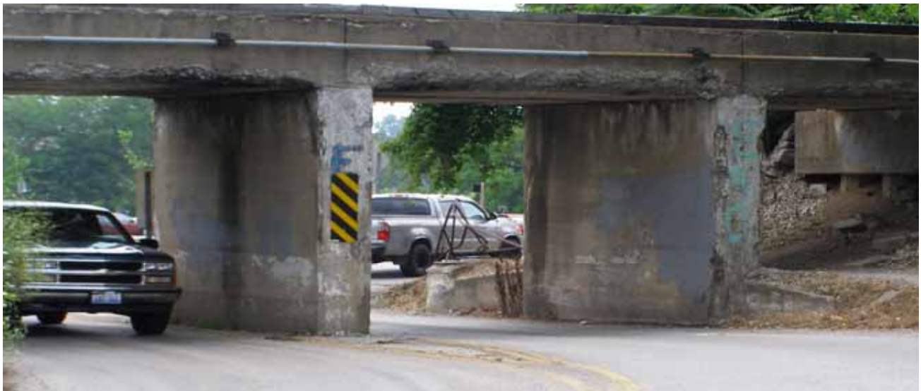
Figure C.17: Image of the existing railroad underpass.
